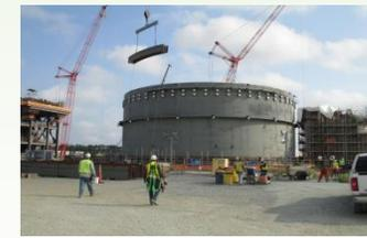
*Placement of Unit 2 CA01 module; progress on Unit 2 shield building (Courtesy of SCANA)*
