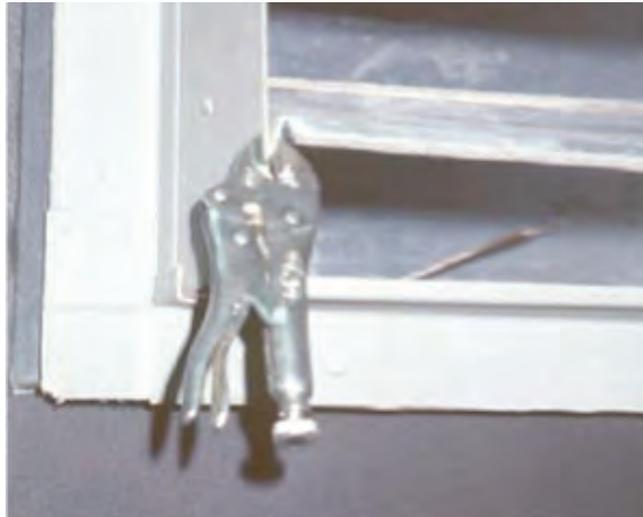
**Figure 9.7.2.** Damper quick fix – not recommended
