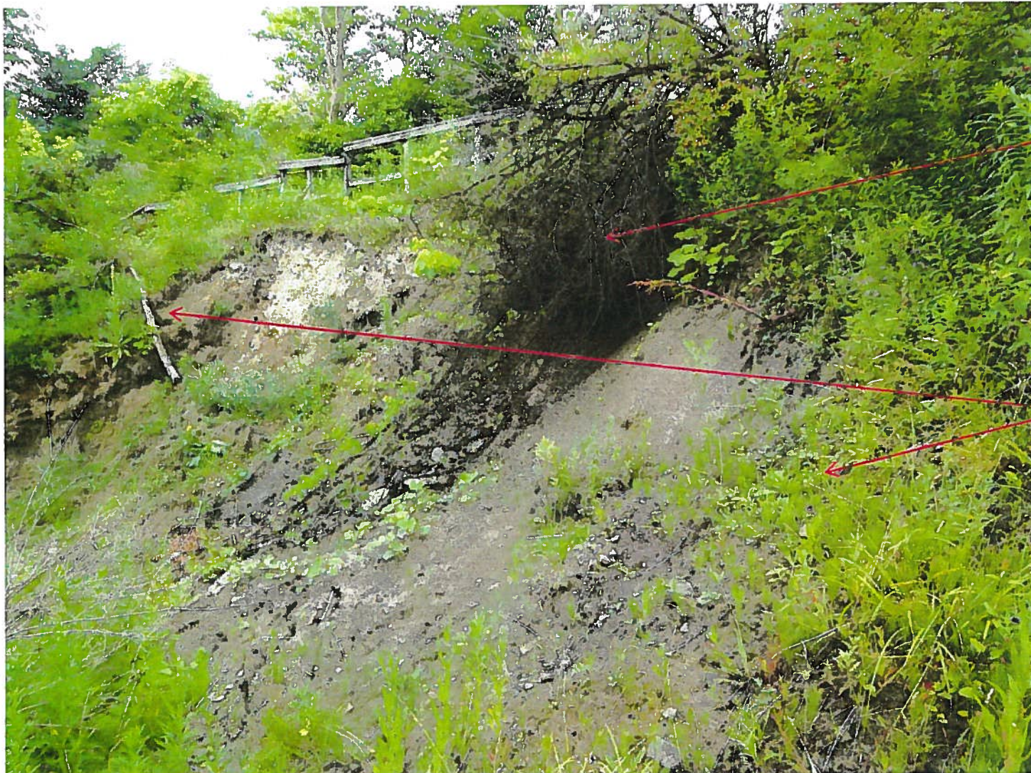
Figure 5. Extent of erosion of the Lagoon 3 embankment at storm water outfall S-09.
