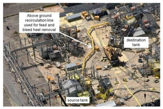
Figure 5.2-3. Above-grade shielded line transfers clarified liquid (2010)
