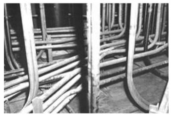
Figure 3.2-1. Tank 4 cooling coils (1953 Pre-Operation)
