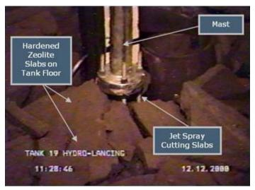
**Figure 5.2-4.** Tank 19 zeolite blocks being broken up by a high pressure hydro-lance
