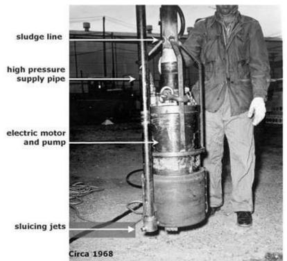
of water to suspend the sludge for a sufficient time to allow the slurry to be pumped from the tank.<sup>13</sup>
