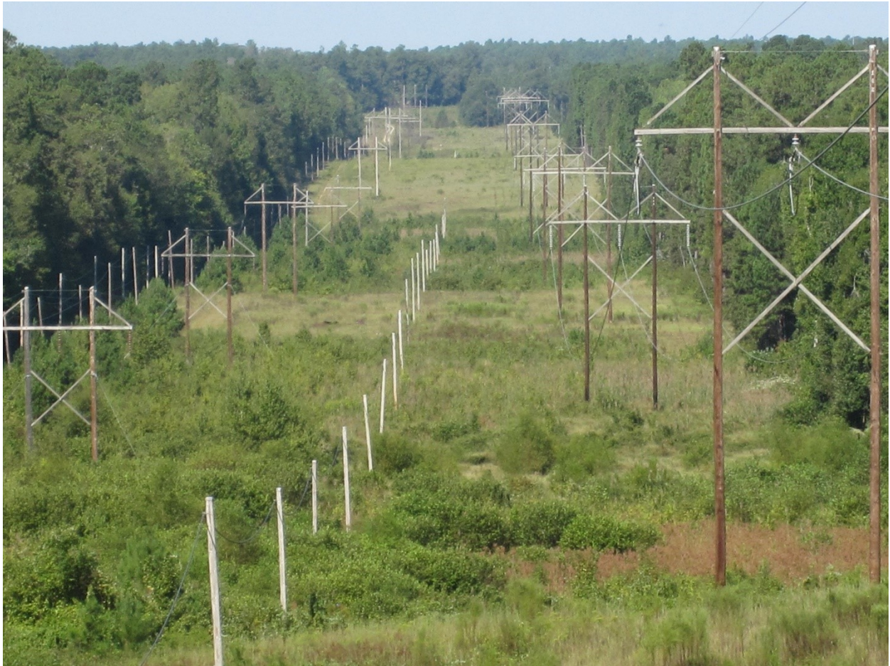
Photograph 2. Typical large wetland crossing of an active 230-kV transmission line(right) and an abandoned 115-kV r/w (left); the length of the crossing is approximately 0.9 mile.
