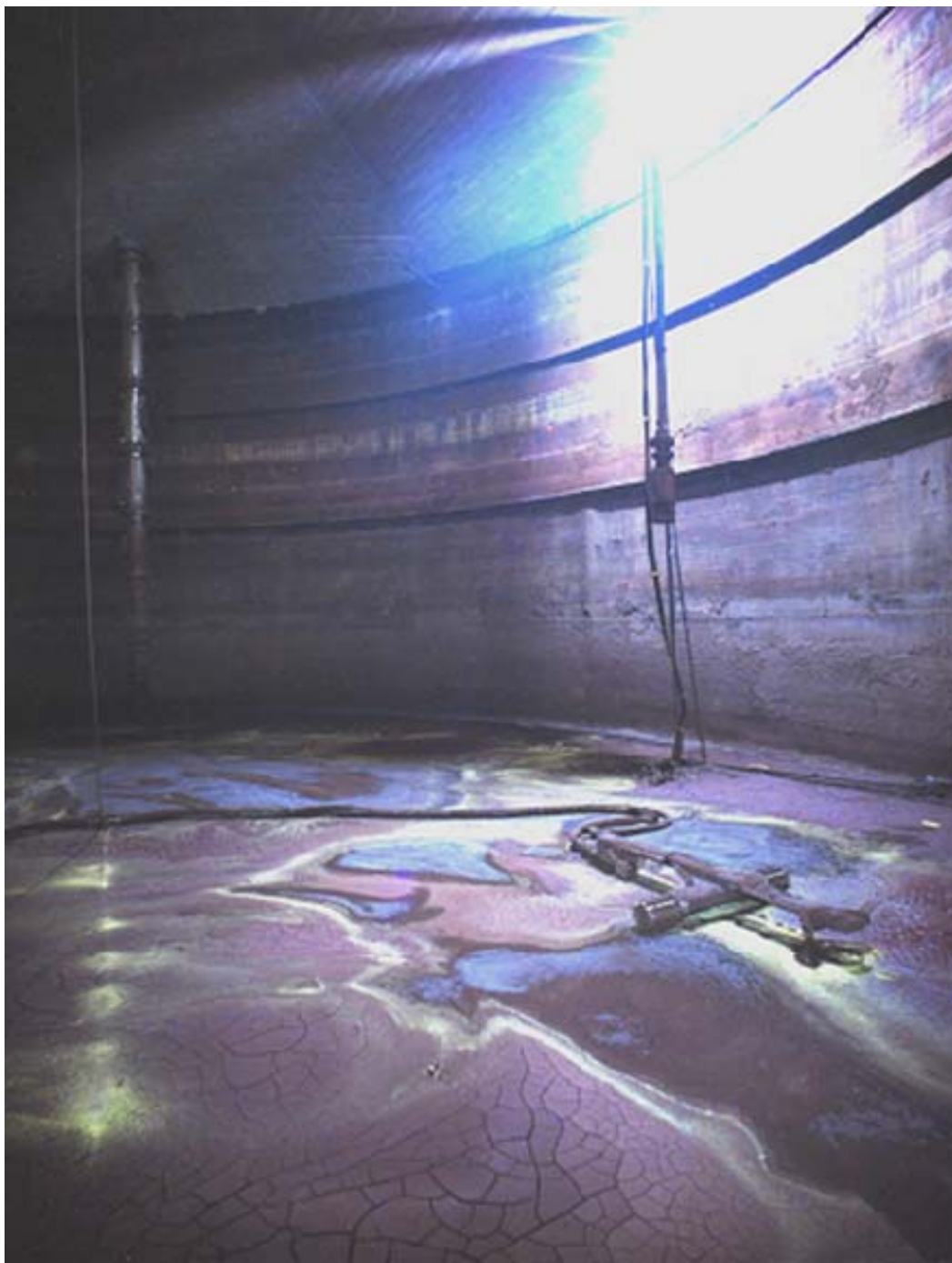
Figure 9.0-3: Tank 18 after Completion of Mantis Operations
