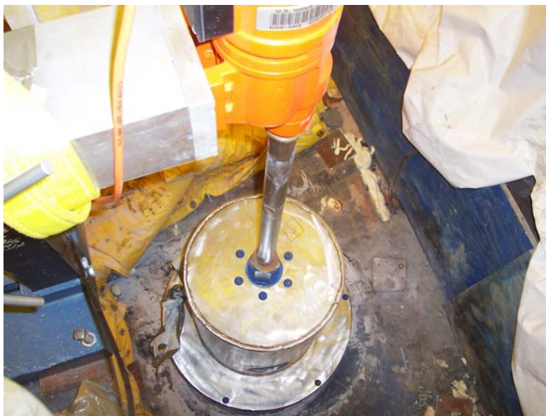
Figure 3.3-15: Core Drilling of New Mechanical Cleaning Riser in Tank 18
