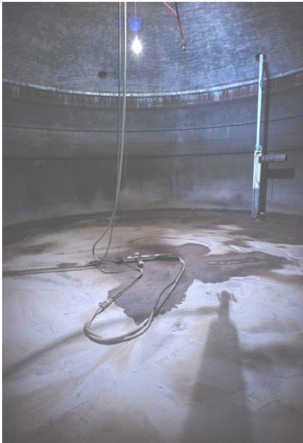
Figure 9.0-4: Tank 19 after Completion of Mantis Operations
