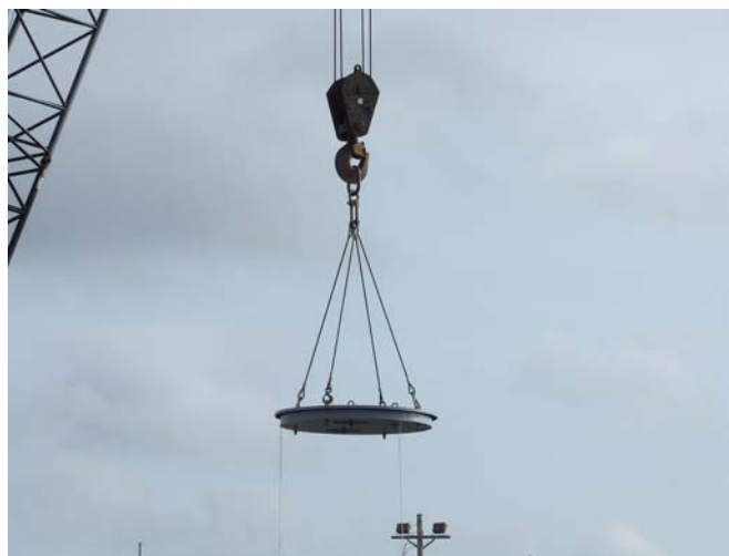
Figure 3.3-9: New Center Riser Cover Being Lowered onto Tank 19
