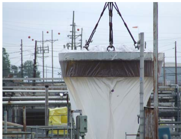
Figure 3.3-8: Removal of the Existing Tank 19 Center Riser Plug
