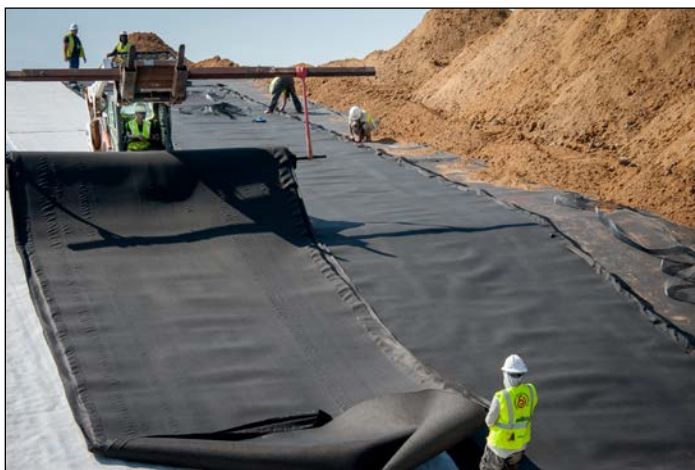
Construction of the Multi-Layer Protective Landfill Cover at the D-Area Ash Basin
