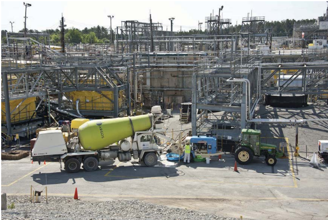
Figure 3-1 SRS Workers Pump Grout from a Concrete Mix Truck to Tank 18F.
