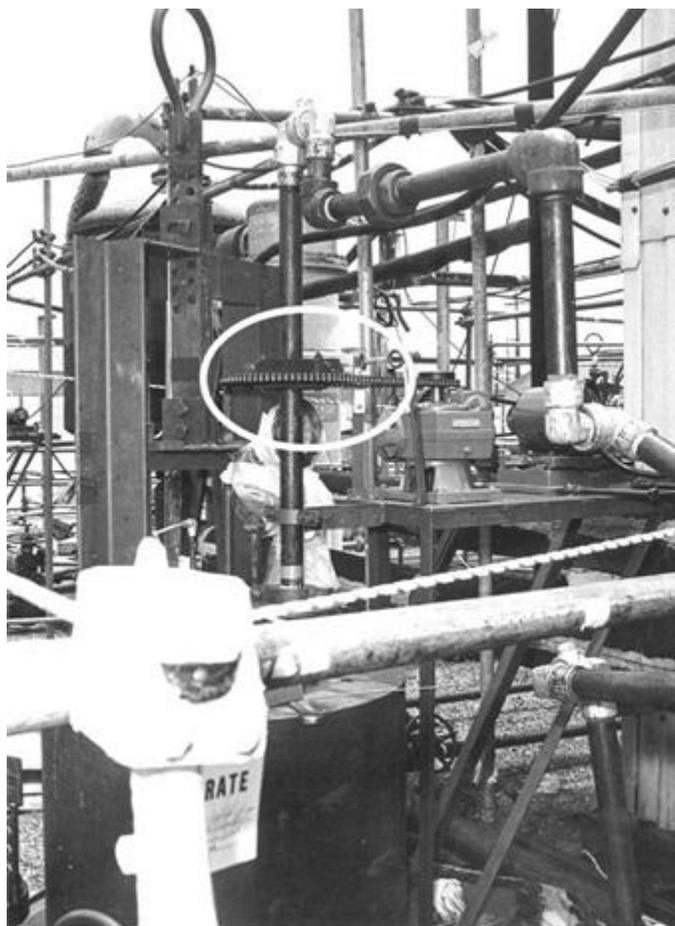
**Figure 5.1-4:** High-pressure line rotated with chain drive (circa 1968)
