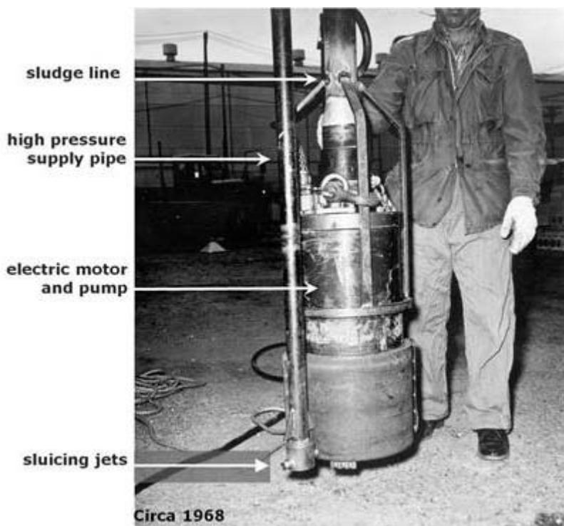
**Figure 5.1-3.** Type I waste tank sludge removal rig before being installed in the tank
