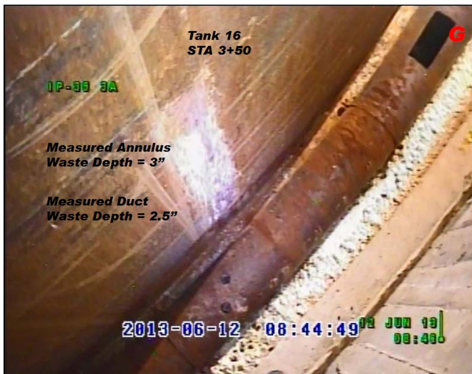
Figure 3.3-3: View of the Tank 16H Annulus during Sampling at IP-35
