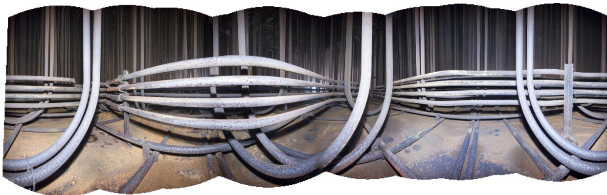
Figure 9.0-1: View of the Tank 16H Primary Tank After Waste Removal
