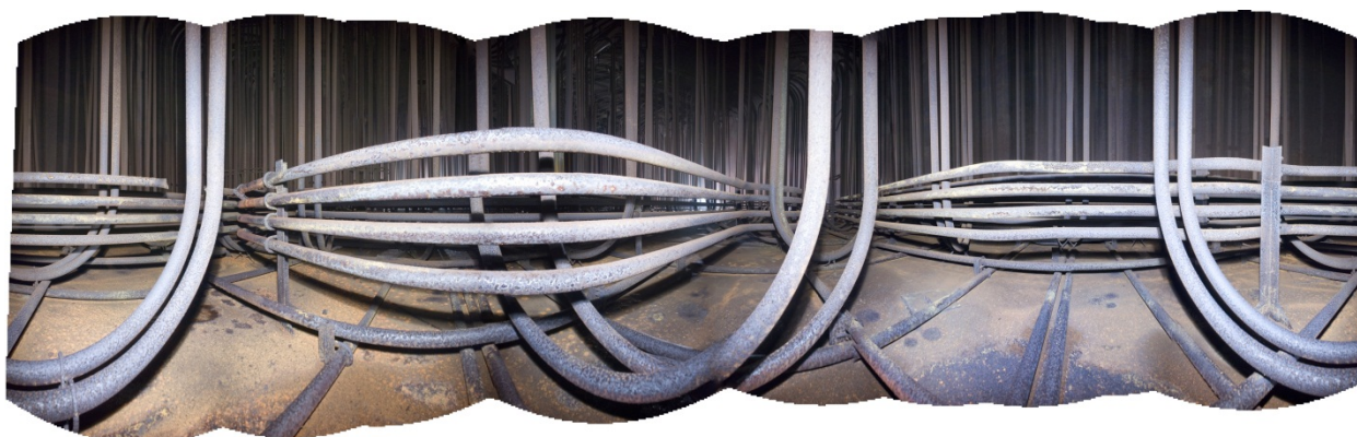
Figure 3.3-1: View of the Tank 16H Primary Tank After Waste Removal
