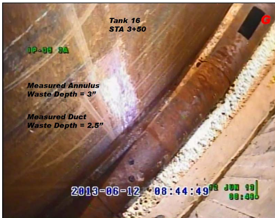
Figure 9.0-2: View of the Tank 16H Annulus during Sampling at IP-35
