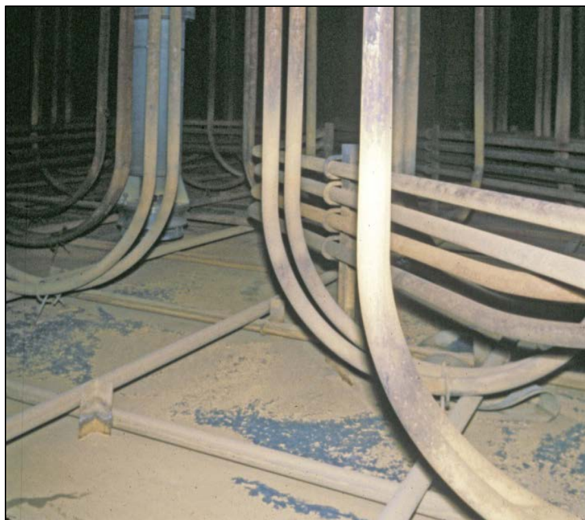
Figure 3.1-14: Photograph of Tank 16H Primary Tank Post Phase 4 Cleaning (December 1980)
