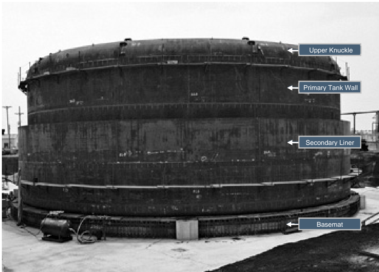
Figure 2.1-45: Typical Type IIIA Tank Primary Tank and Secondary Liner - Late Construction (Vault Wall Not Constructed)
