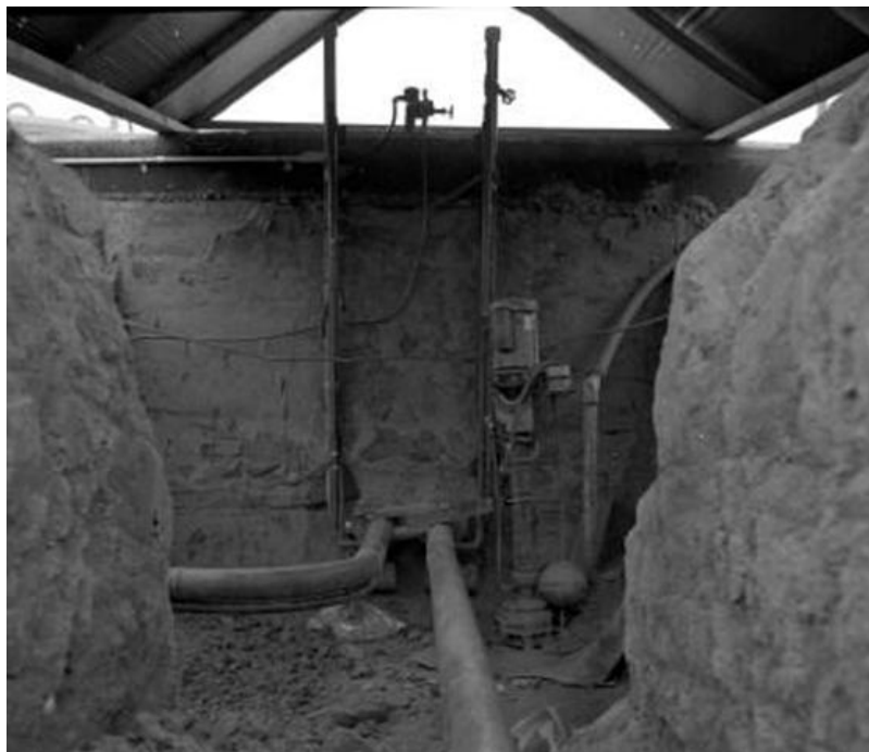
Figure 2.1-57: HTF Waste Tank Transfer Line During Construction
