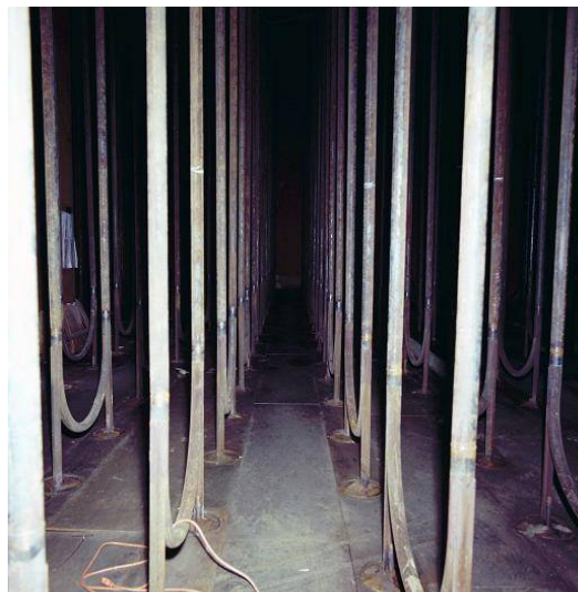
Figure 2.1-48: Typical Type IIIA Tank Cooling Coils During Construction
