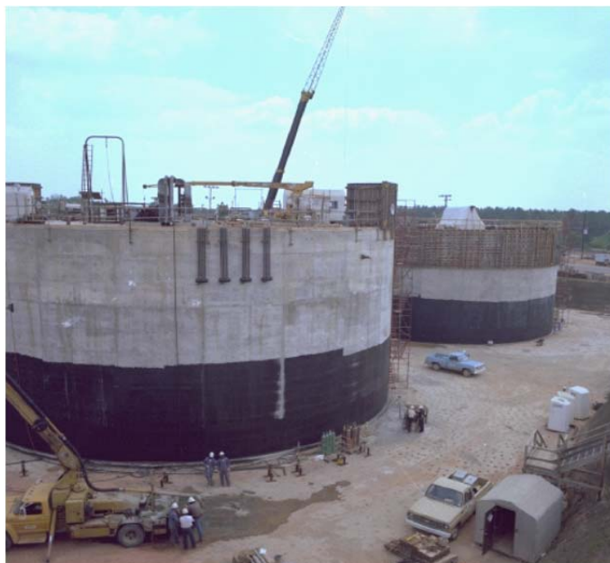
Figure A.2-1: Waste Tanks Under Construction
