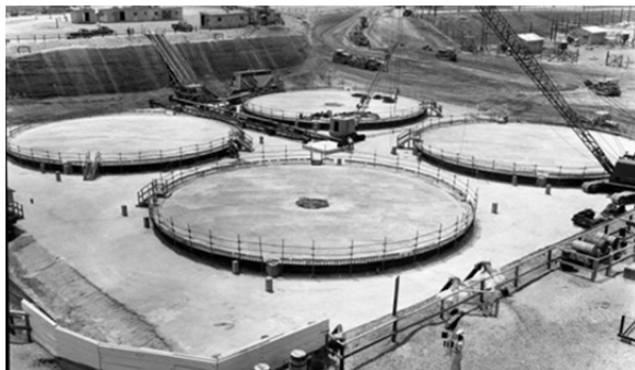
Figure 2.1-36: Type II Tank Basemat Construction
