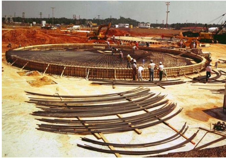
Figure 2.1-44: Typical Type III/IIIA Tank Basemat Construction
