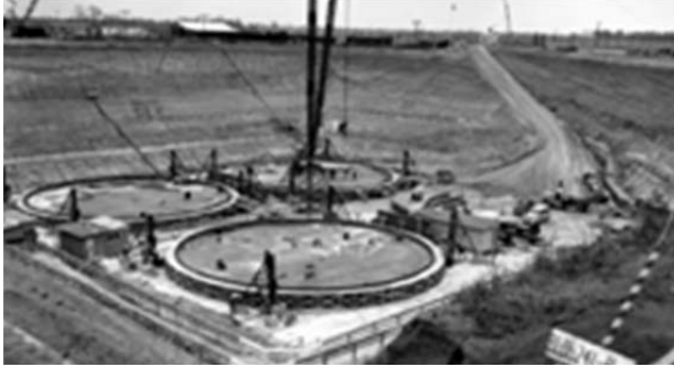
Figure 2.1-30: Type I Tank Basemat Construction
