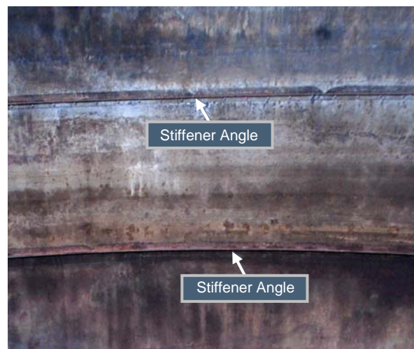
Figure 2.1-45: Typical Type IV Waste Tank Stiffener Angles
