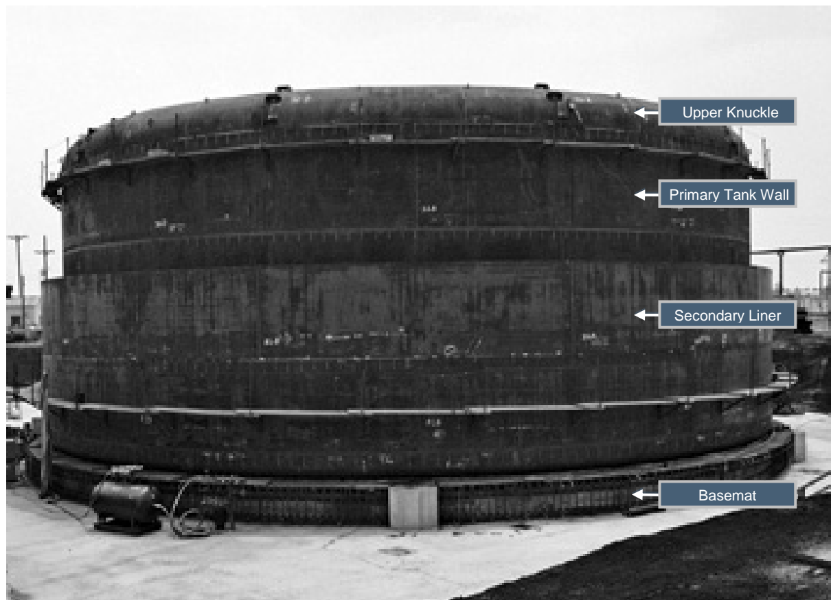
Figure 2.1-38: Typical Type IIIA Waste Tank Primary Tank and Secondary Liner - Late Construction (Vault Wall Not Constructed)
