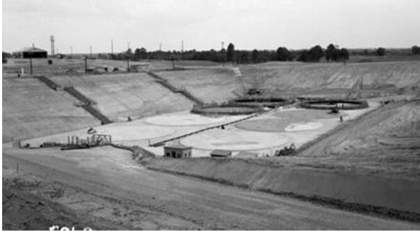
Figure 2.1-30: Type I Waste Tank Basemat Construction
