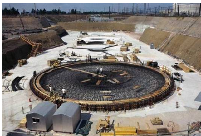
Figure 2.1-37: Typical Type III/IIIA Waste Tank Basemat Construction
