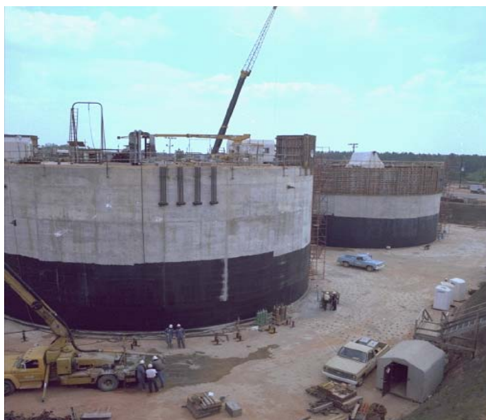
Figure A.2-1: Waste Tanks Under Construction
