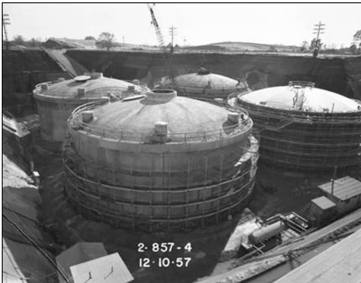
Figure 2-5: Type IV Tanks Under Construction
