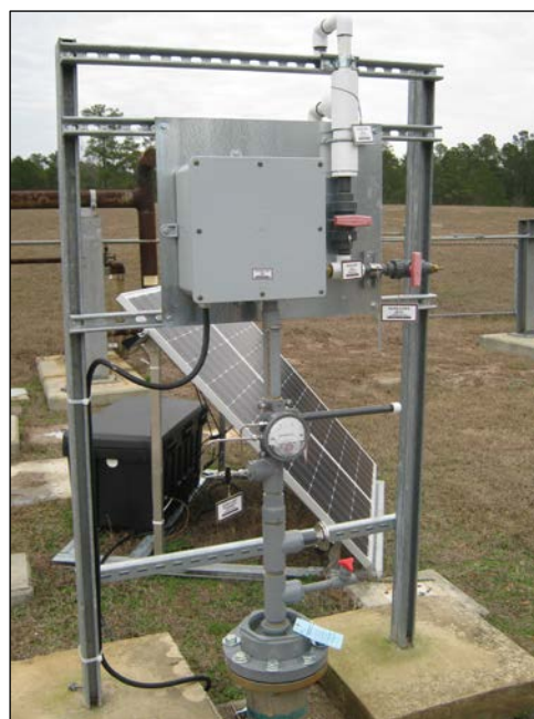
A MicroBlower Pumps Volatile Organic Contaminants from the Subsurface
