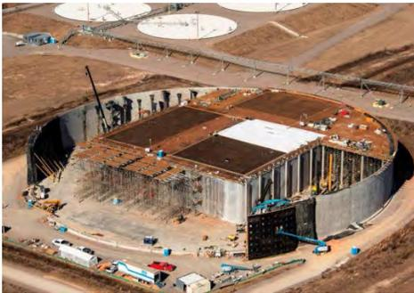
**In 2014, Construction Continued on SRS's First Mega-Volume Saltstone Disposal Unit (SDU), Capable of Holding 10 times the Volume of Waste in Current SDUs**
