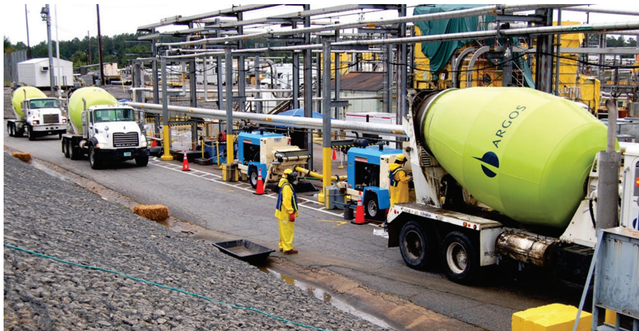
Figure 3-1 SRS Employees Grouting Tanks 5F and 6F
