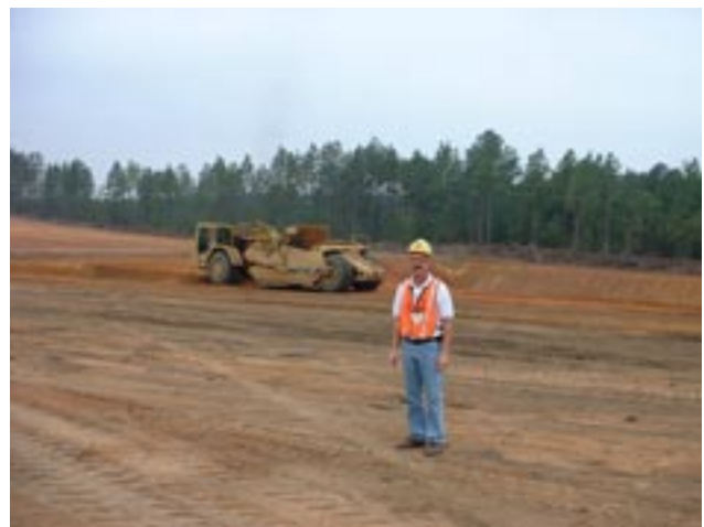
Following timely completion of the EA and FONSI, site clearing began at the borrow pit site.
