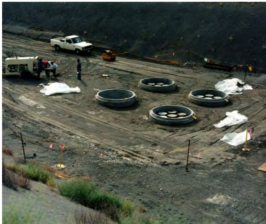
Figure 2.13. High-Integrity Containers in a Low-Level Waste Disposal Trench
