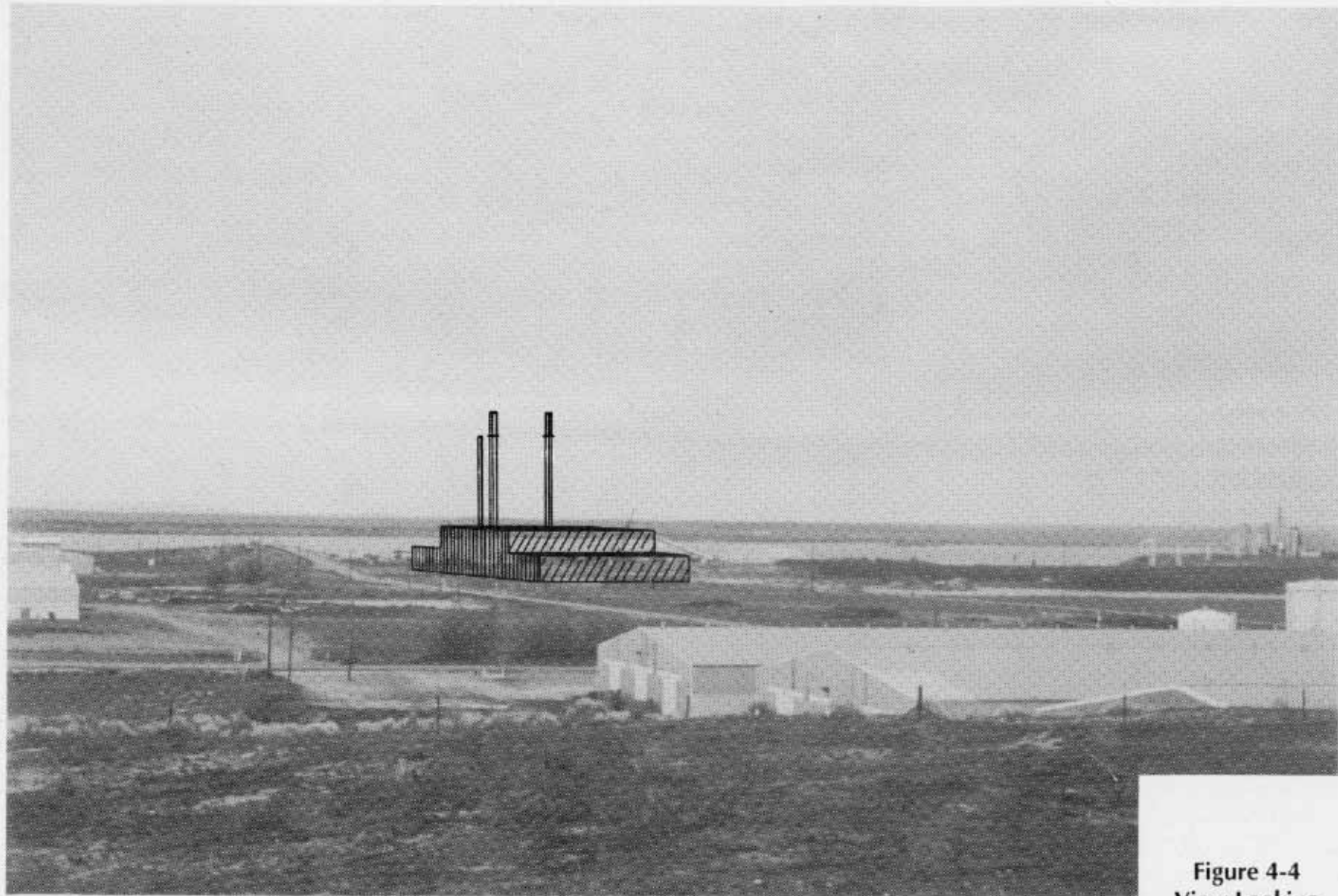
Coyote Springs Cogeneration Plant - Morrow County, Oregon
