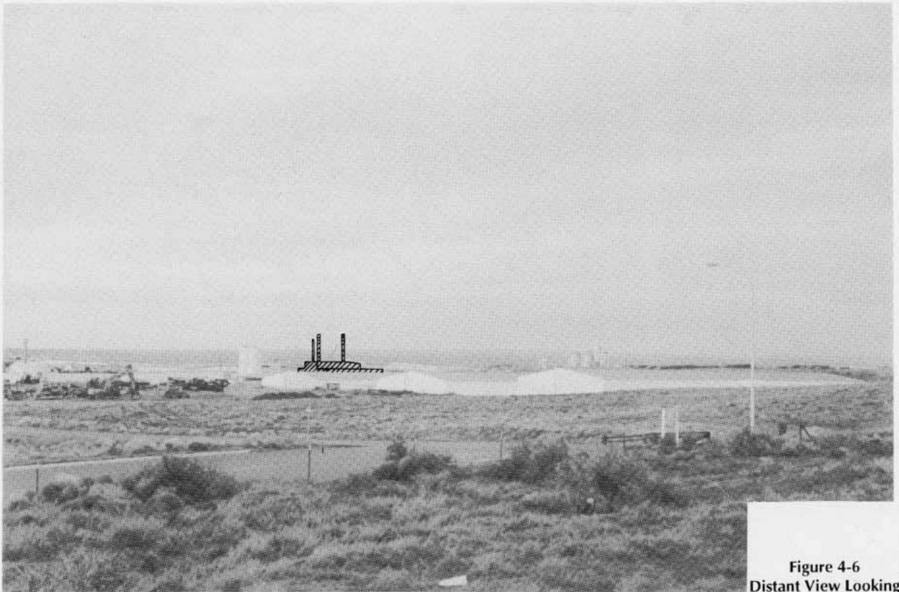
Coyote Springs Cogeneration Plant - Morrow County, Oregon
