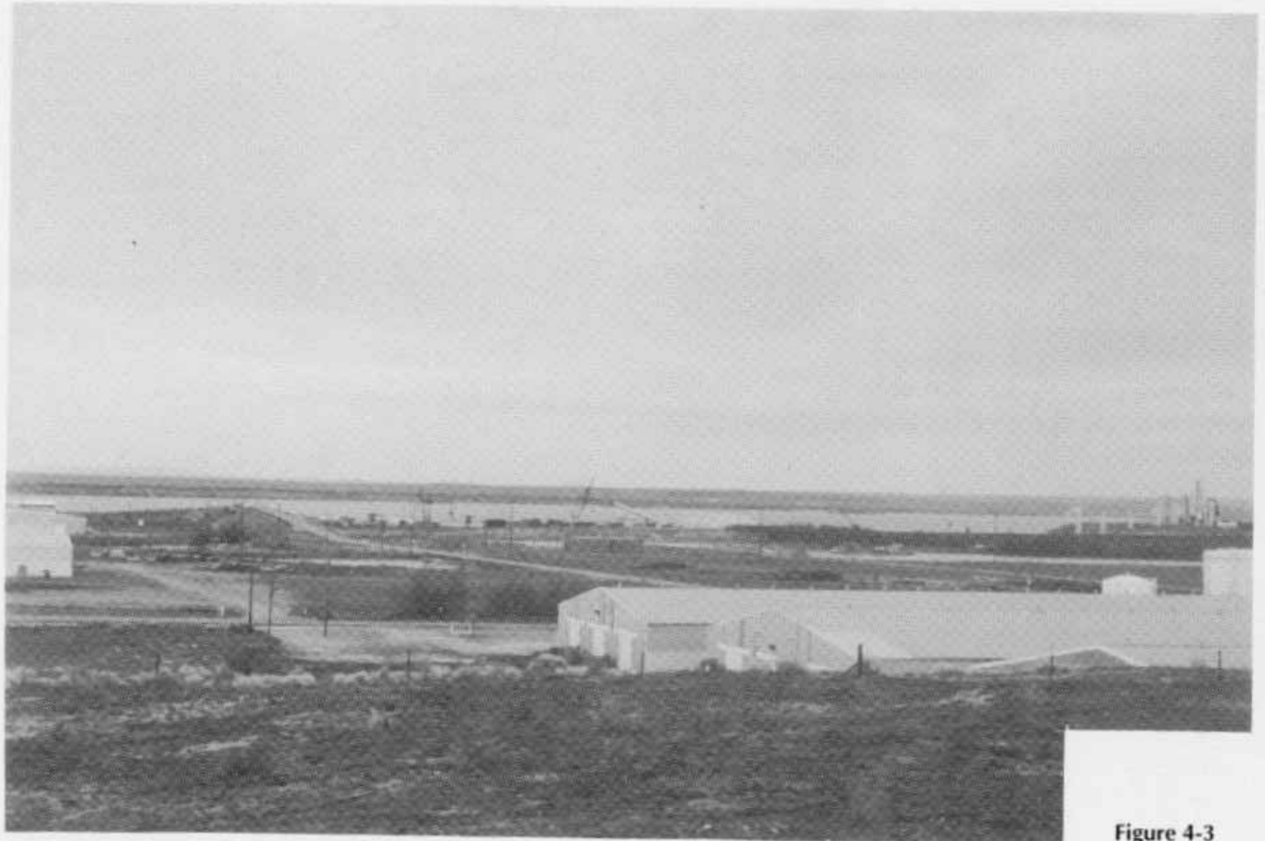
Coyote Springs Cogeneration Plant - Morrow County, Oregon
