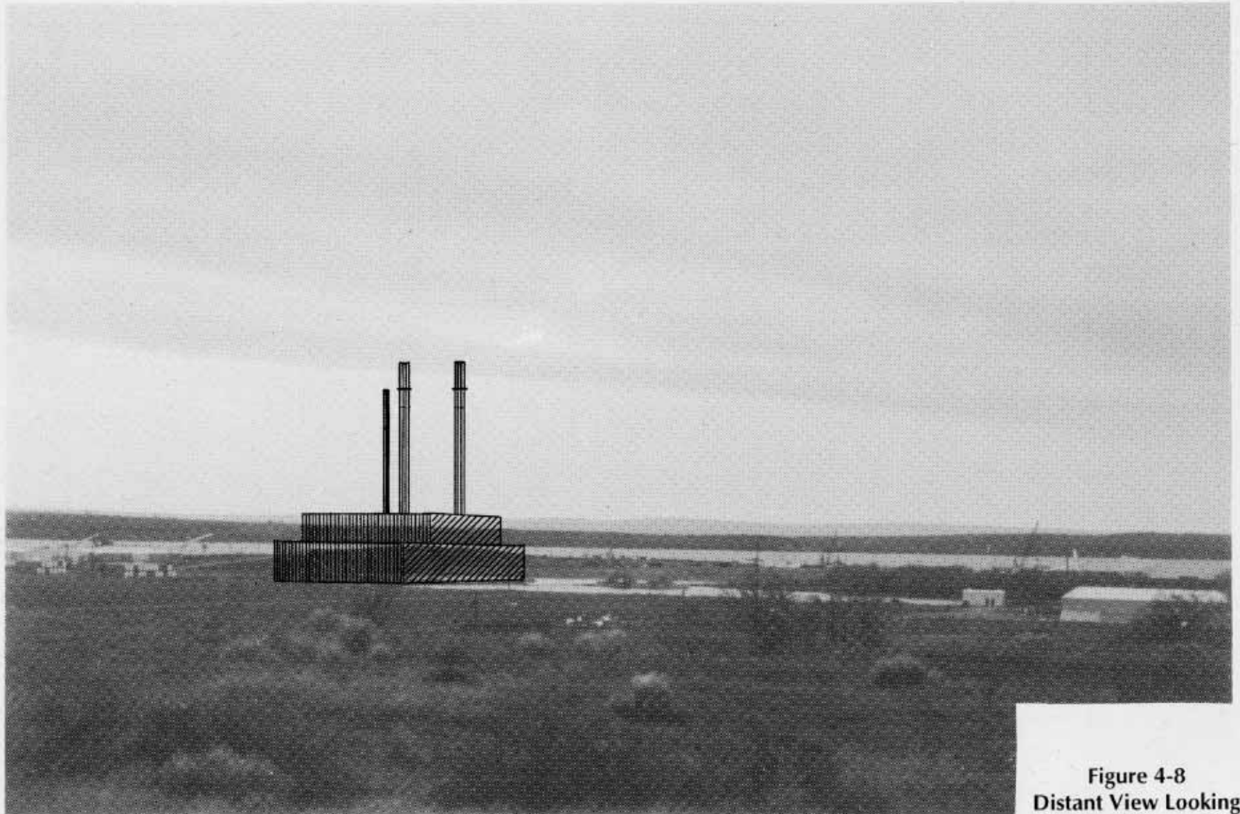
Coyote Springs Cogeneration Plant - Morrow County, Oregon
