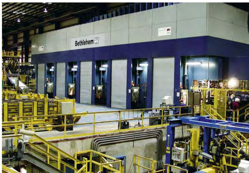
Figure 2.5: Typical Modern PLTCM While Operating
