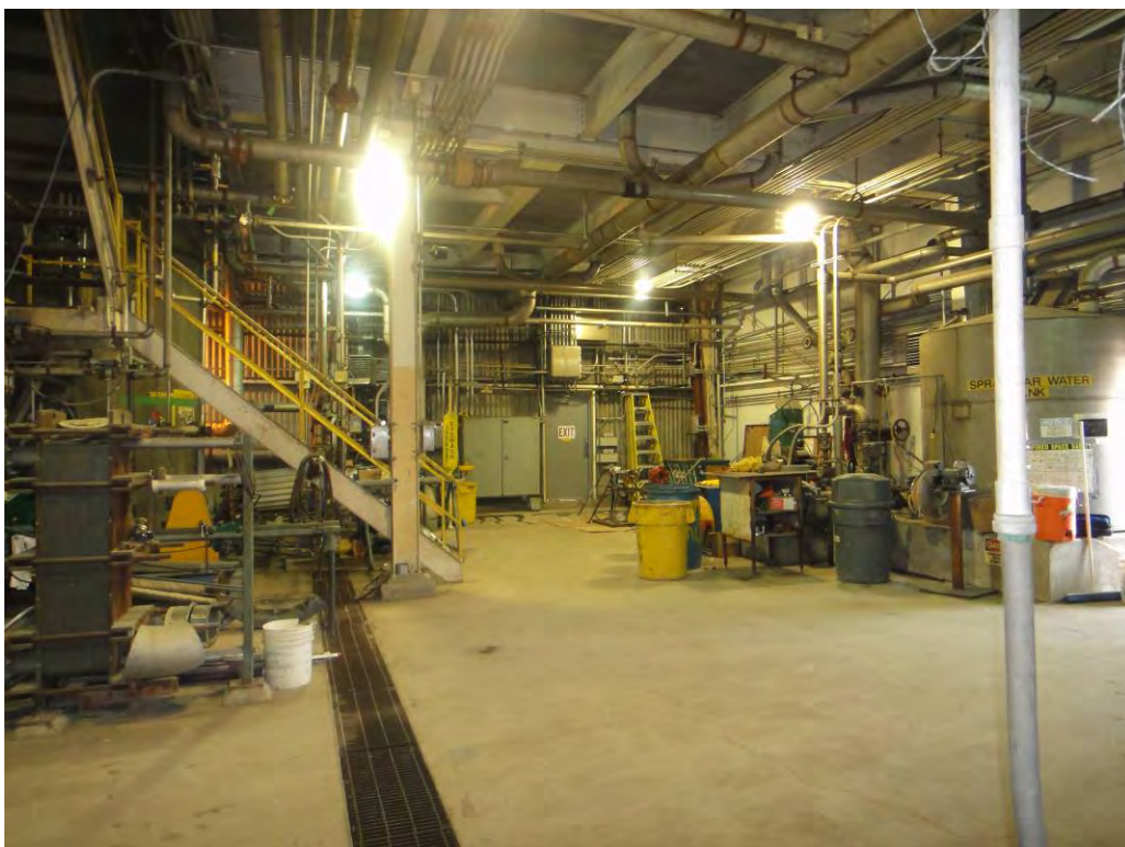
Figure 7. Second Interior View of Blower Building
