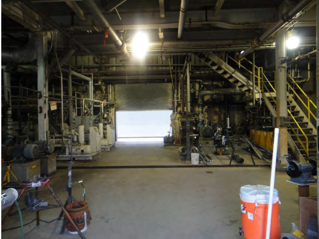
Figure 8. Third Interior View of Blower Building
