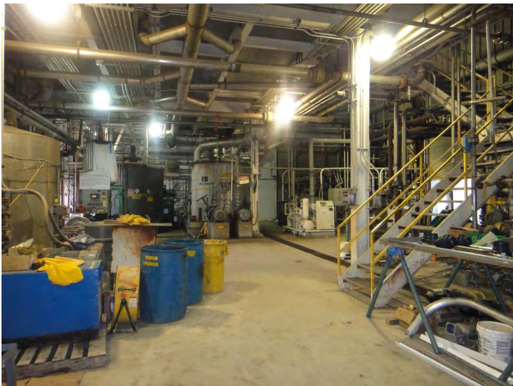
Figure 6. First Interior View of Blower Building
