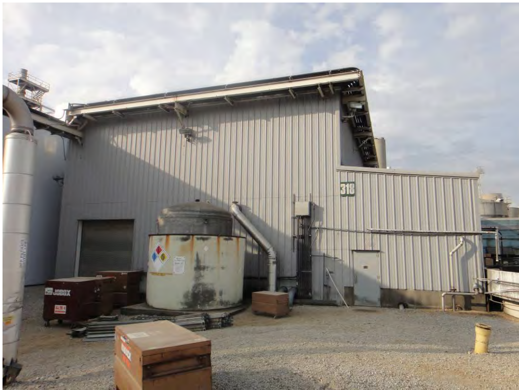
Figure 4. Side Exterior View of Blower Building
