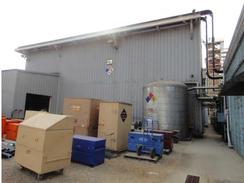
Figure 5. Rear Exterior View of Blower Building
