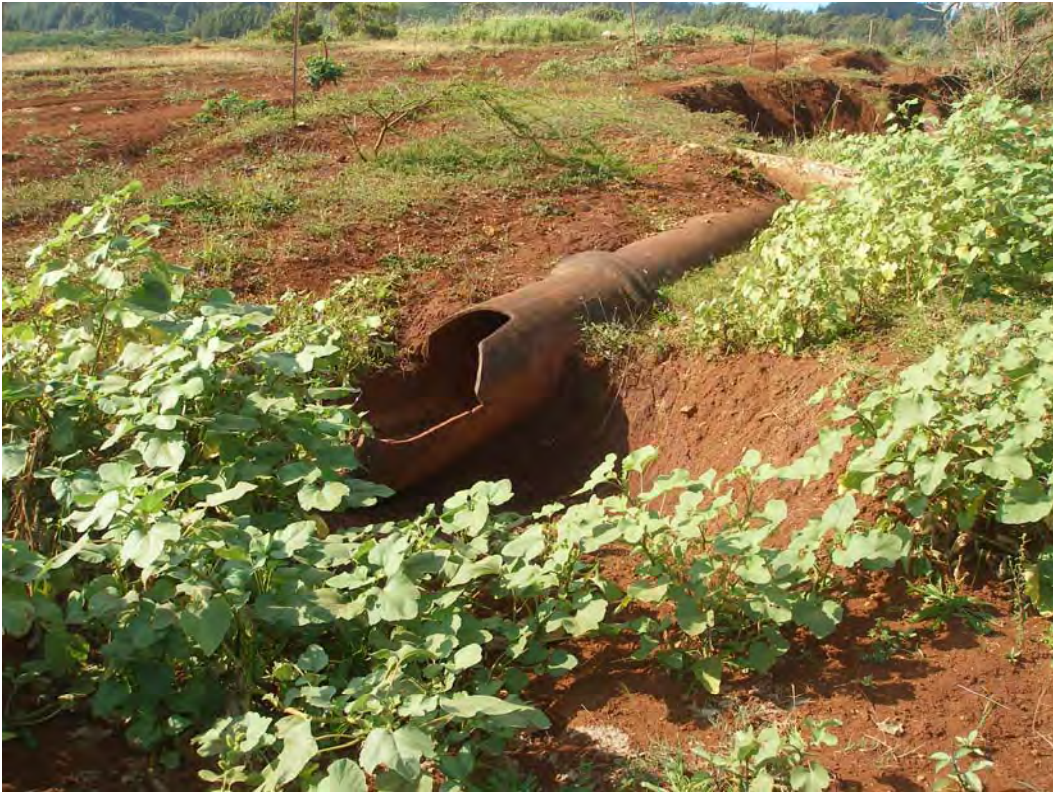
Figure 35. Exposed section of an underground pipe between the reservoir and Pump 18, view to southeast.
