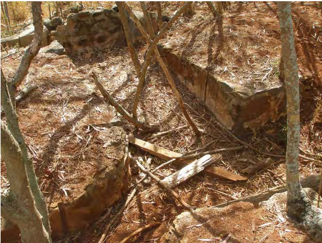
Figure 43. Stone and concrete lined ditch junctions next to the tin shack.
