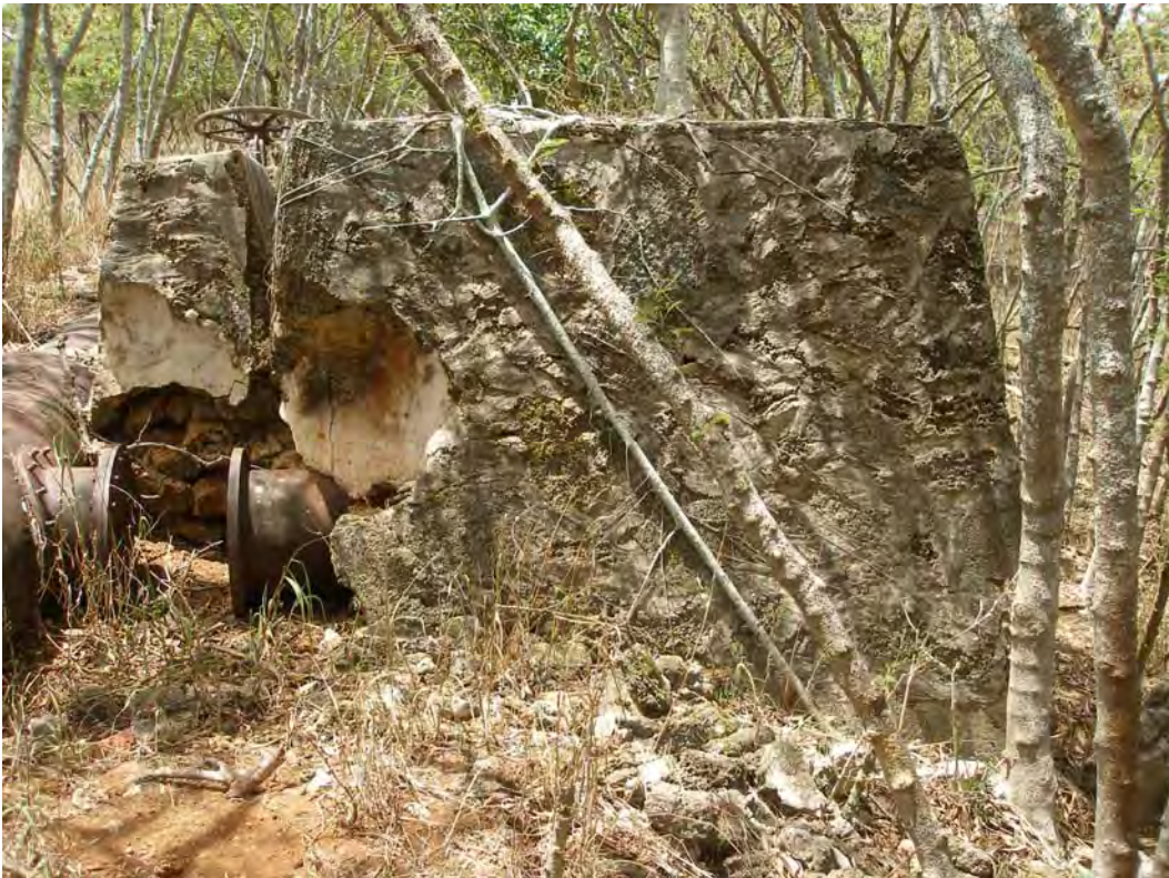
Figure 50. Flume/pipe junction, view to southwest.
