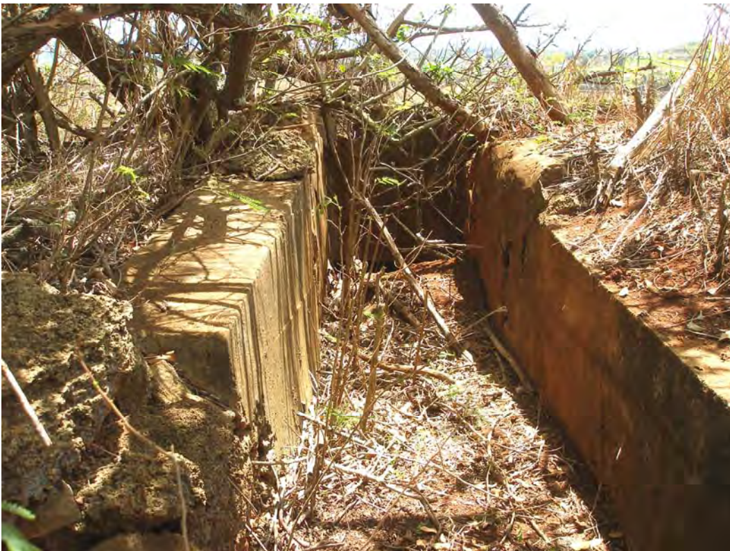
Figure 45. Concrete flume connecting to the underground pipe, view to east.
