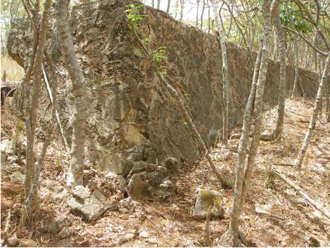
Figure 49. Northern exterior edge of stone and concrete flume, view to northwest.
