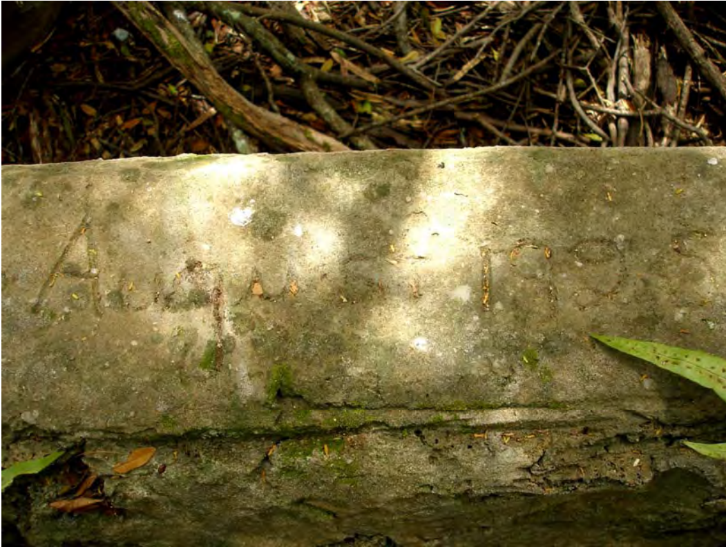
Figure 33. August 1925 inscribed in concrete near the reservoir outflow pipe, over view.
