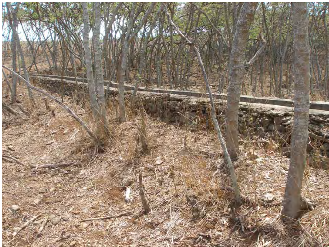
Figure 30. Stone and concrete flume edge.
