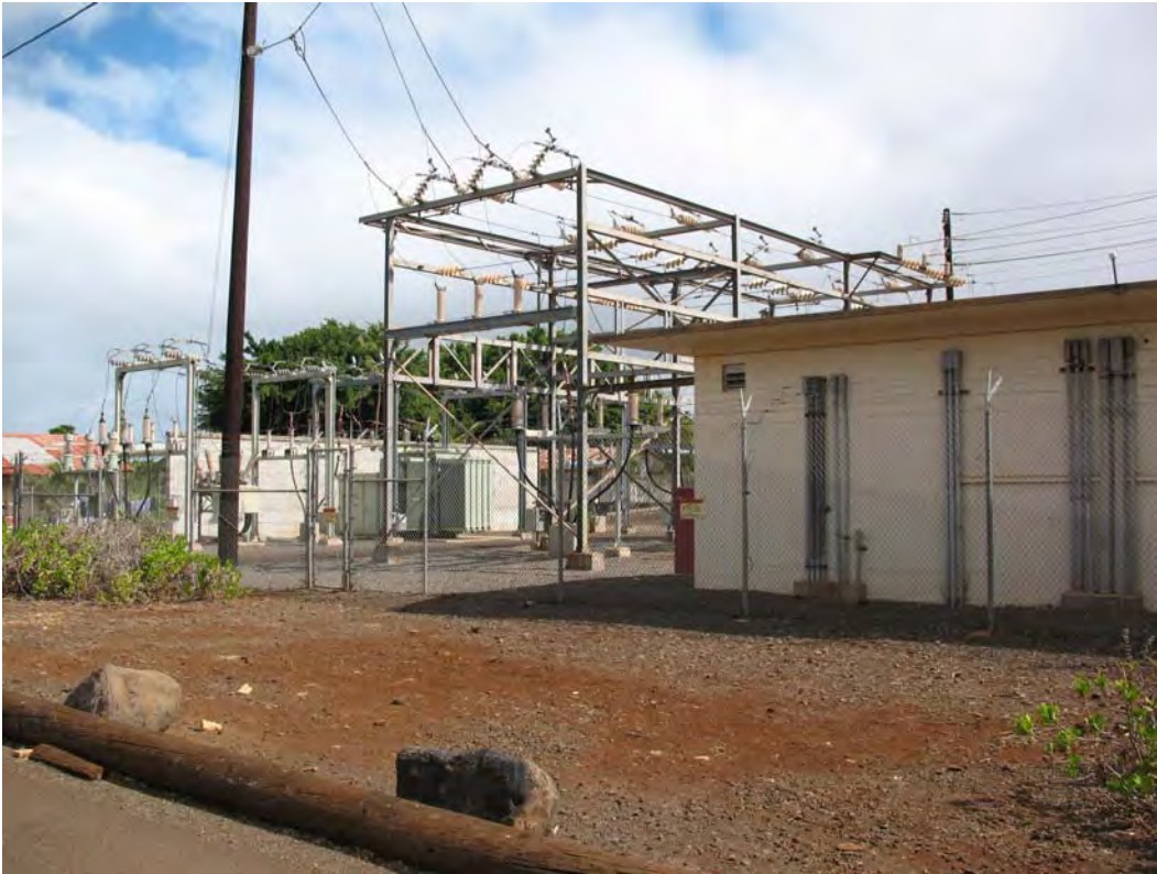
Figure 2. Existing HECO Waialua substation.
