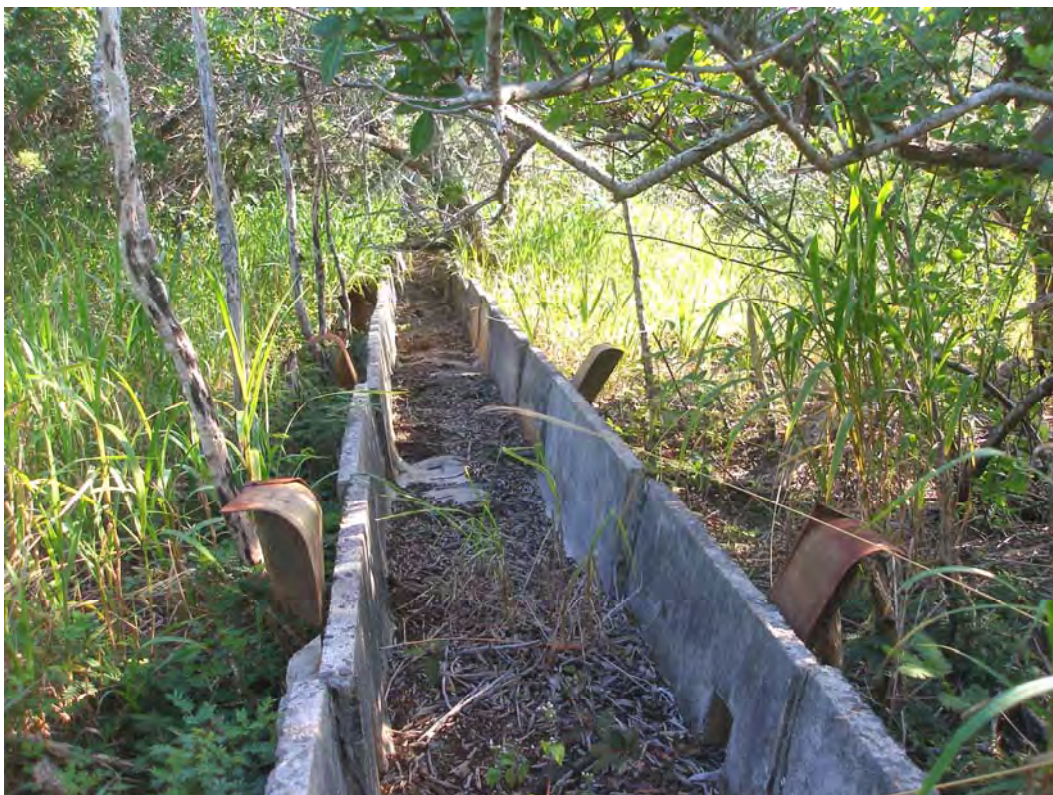
Figure 26. Sectional concrete flume.
