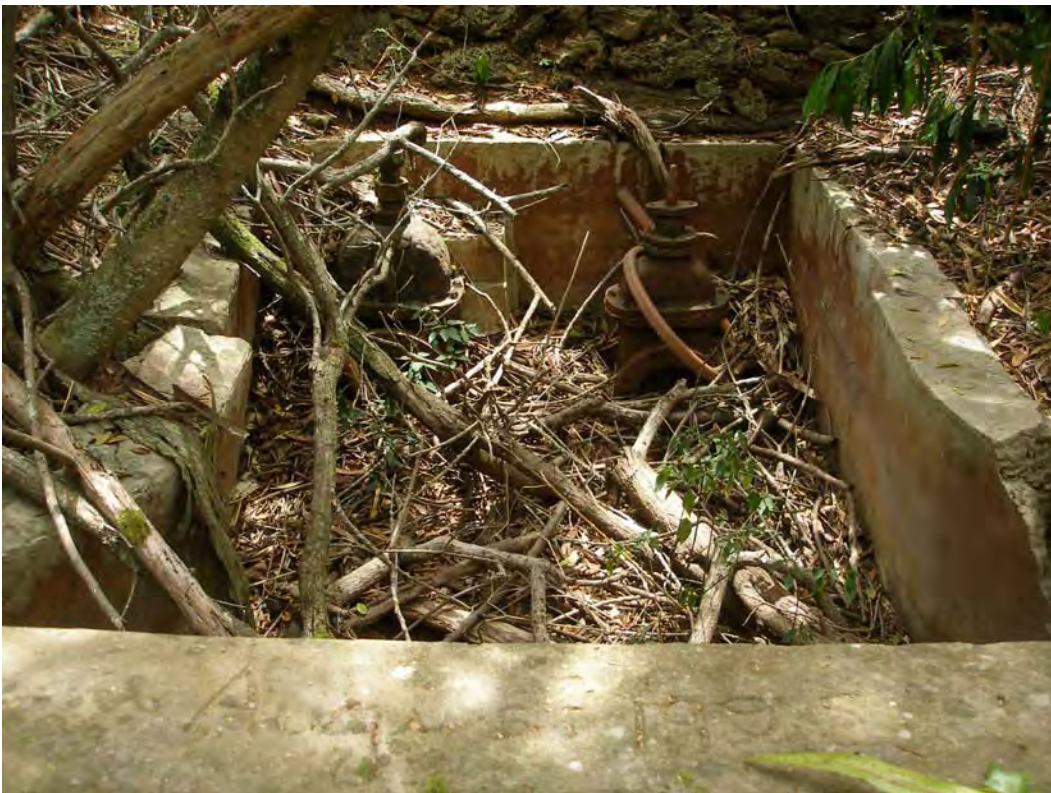
Figure 34. Reservoir outflow pipe, view to east.
