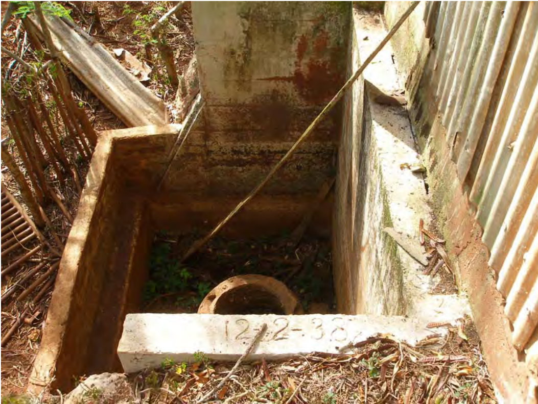
Figure 40. "12-2-38" inscribed in the concrete foundation of a small tin shack pump house near the northwestern boundary of the APE.
