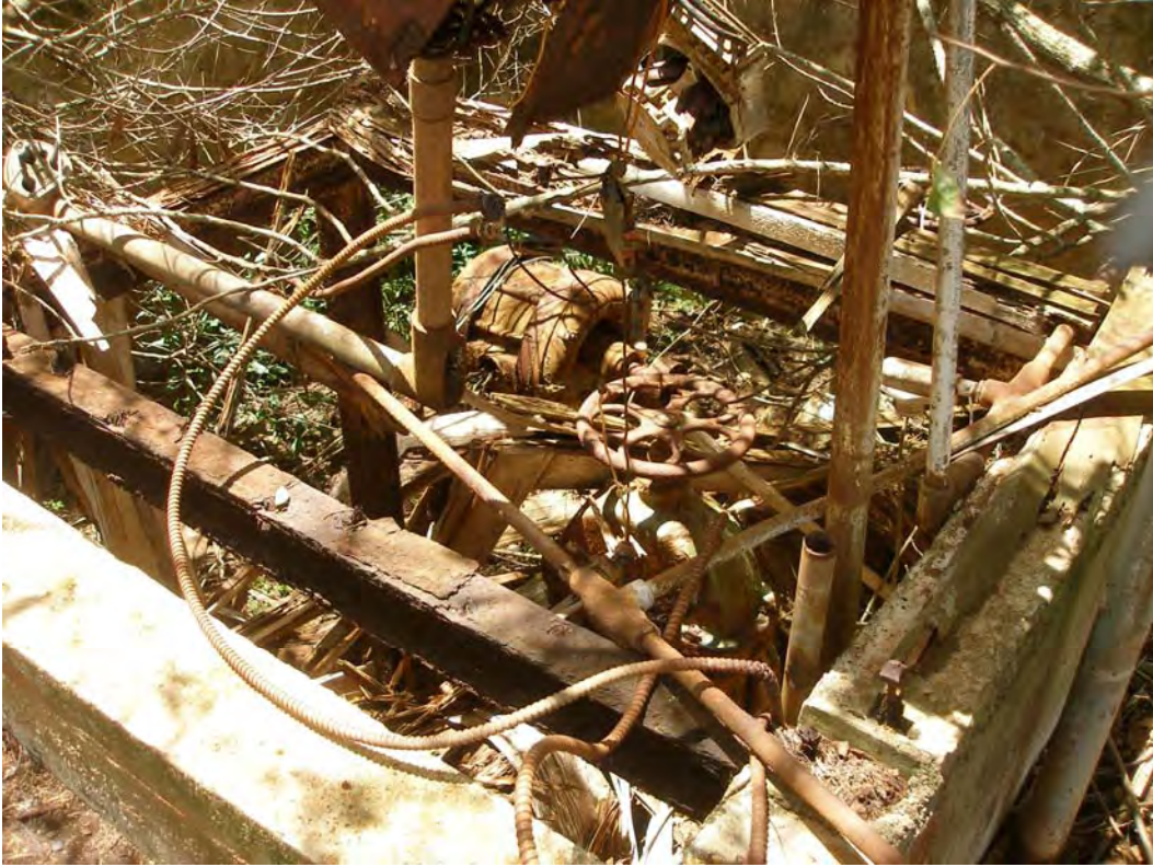
Figure 47. Pump 18 machinery, view to southeast.
