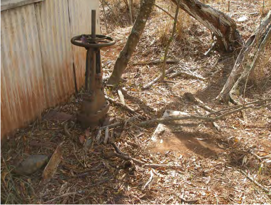
Figure 42. Shut-off valve along the southern edge of the shack, view to east.
