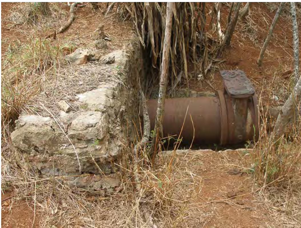
Figure 37. Reservoir inlet pipe/valve, view to east.
