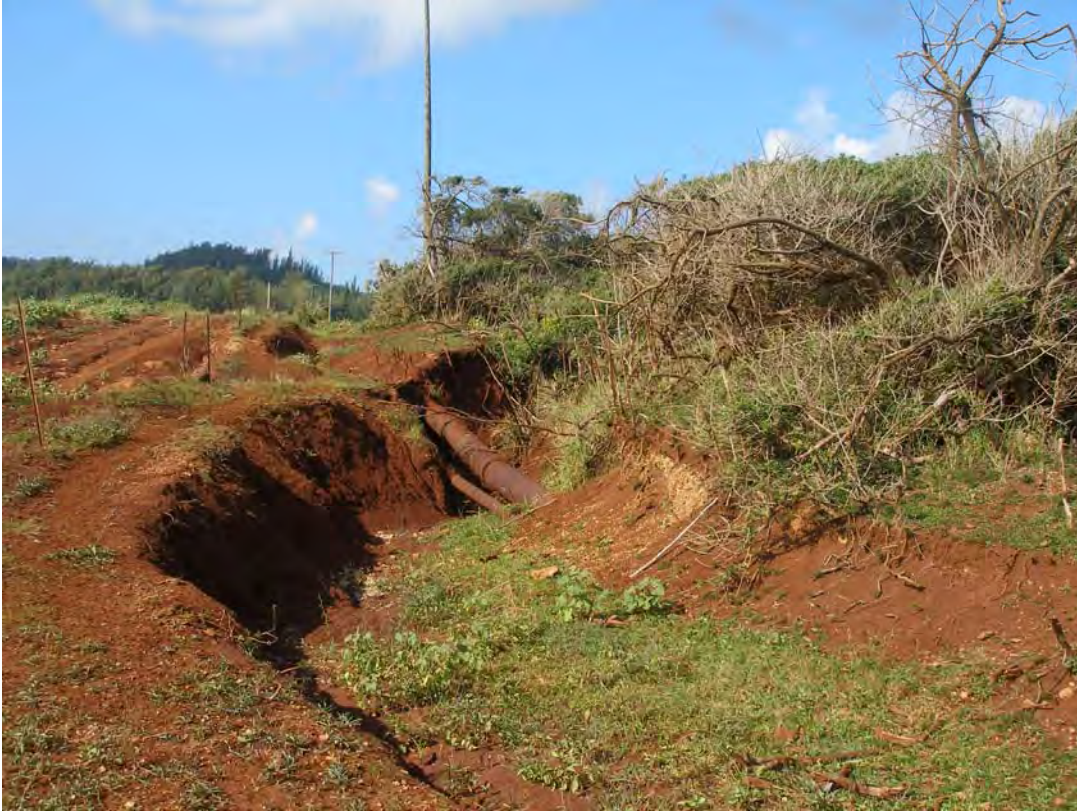
Figure 5. View to south of the “aqueduct” (large metal water pipe line) crossing the project area.
