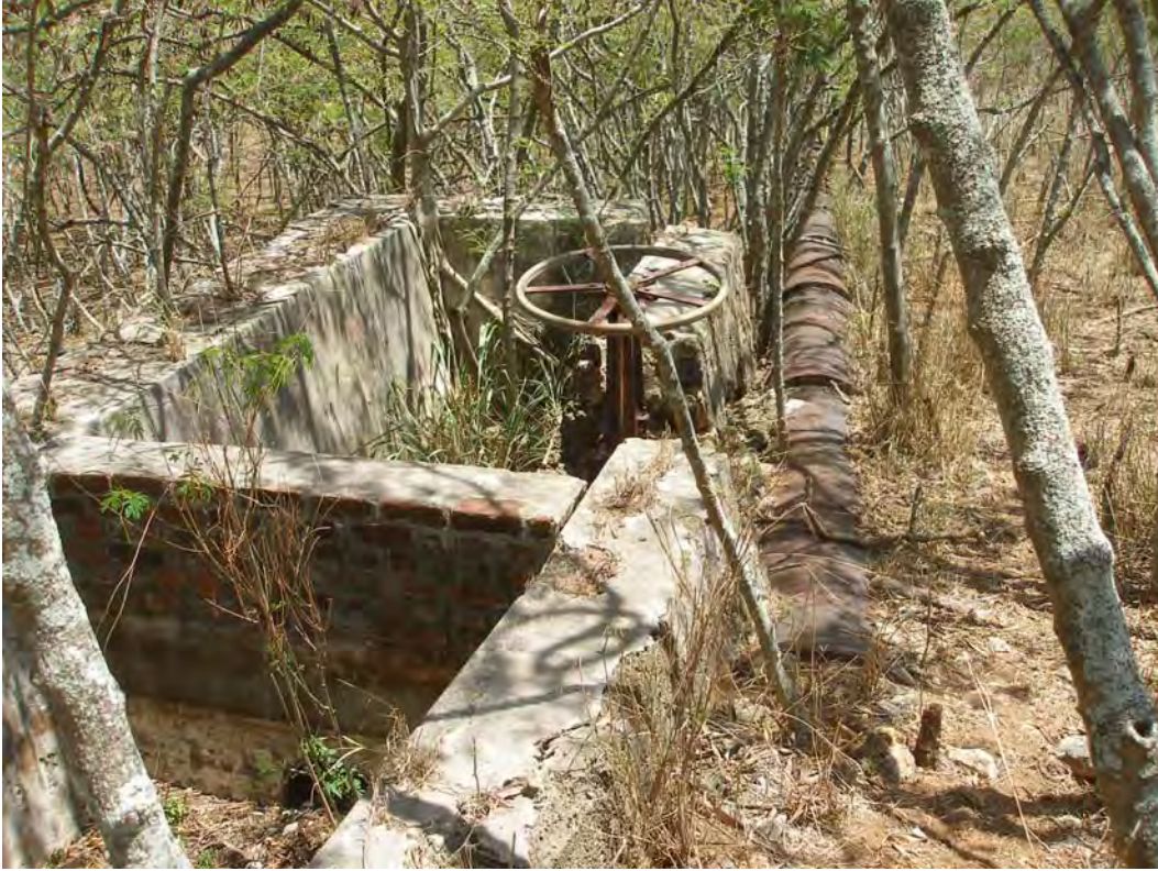
Figure 51. Shut-off valve, view to northeast.
