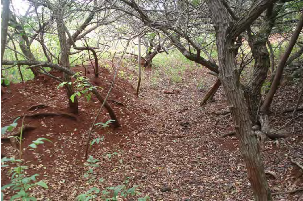
Figure 24. A typical soil berm lined ditch.
