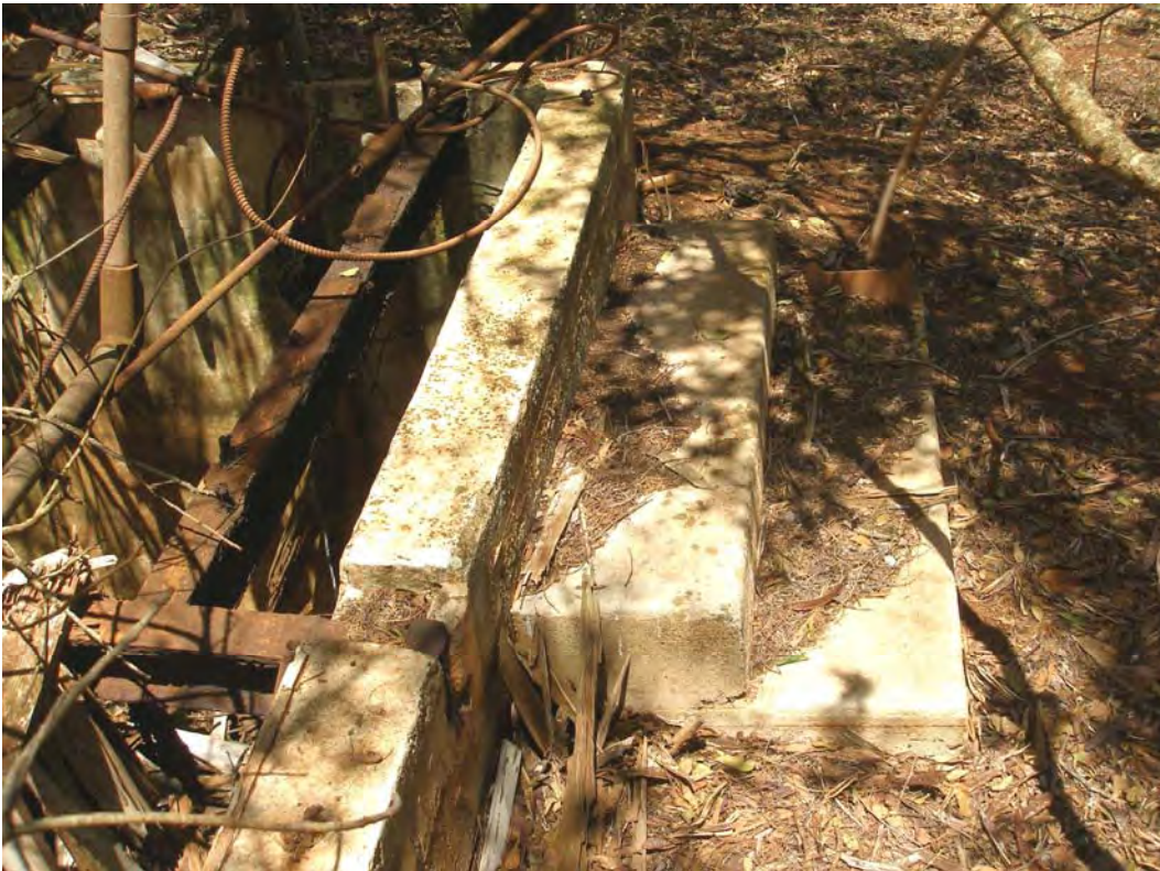
Figure 48. Stairs at Pump 18, view to northwest.
