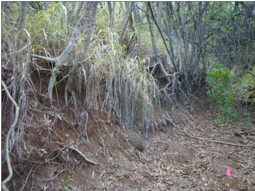
Figure 15. Exposed koa haole tree roots along the elevated banks of Ohia'ai Gulch.
