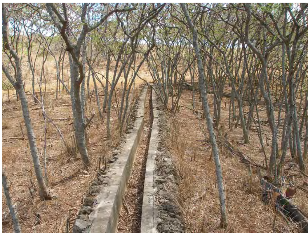
Figure 31. Stone and concrete flume water channel.
