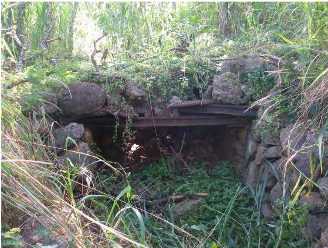
Figure 32. A former bridge crossing an irrigation ditch.
