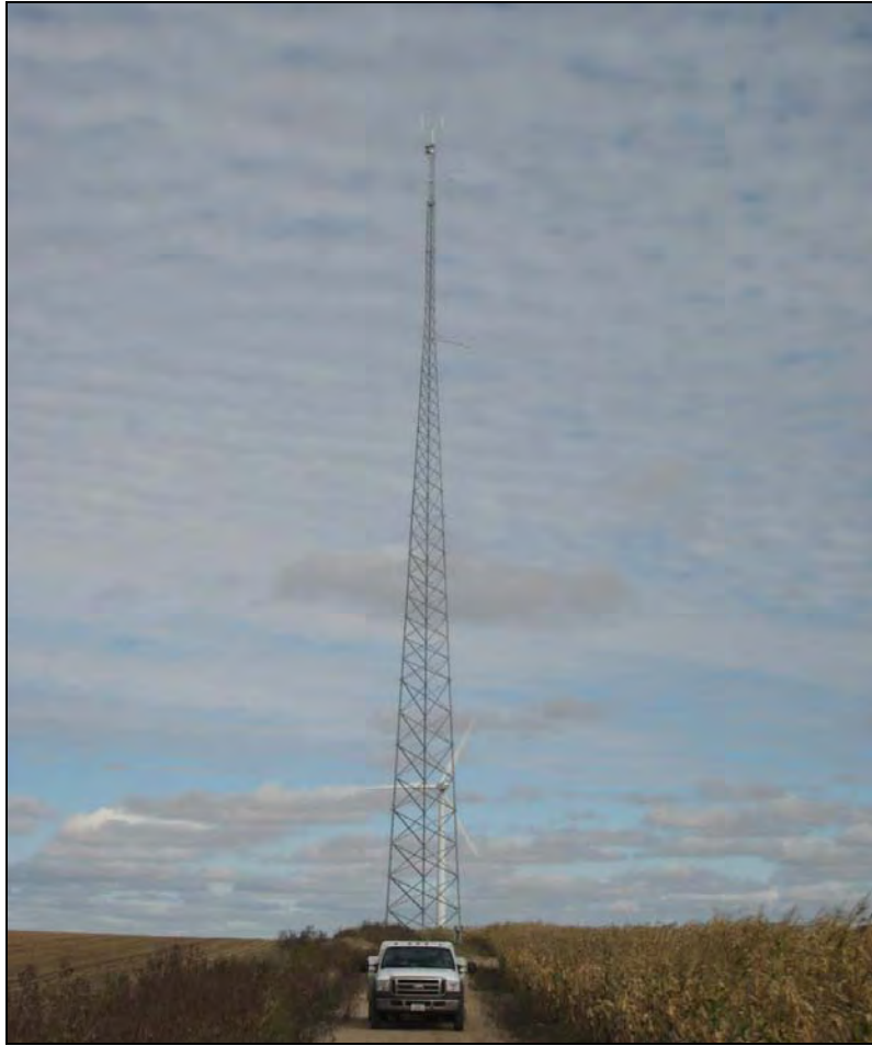
Figure 2-3. Unguyed met tower, approximately 262.5 ft (80 m) tall, similar to the one proposed for the Kahuku Wind Power facility.
