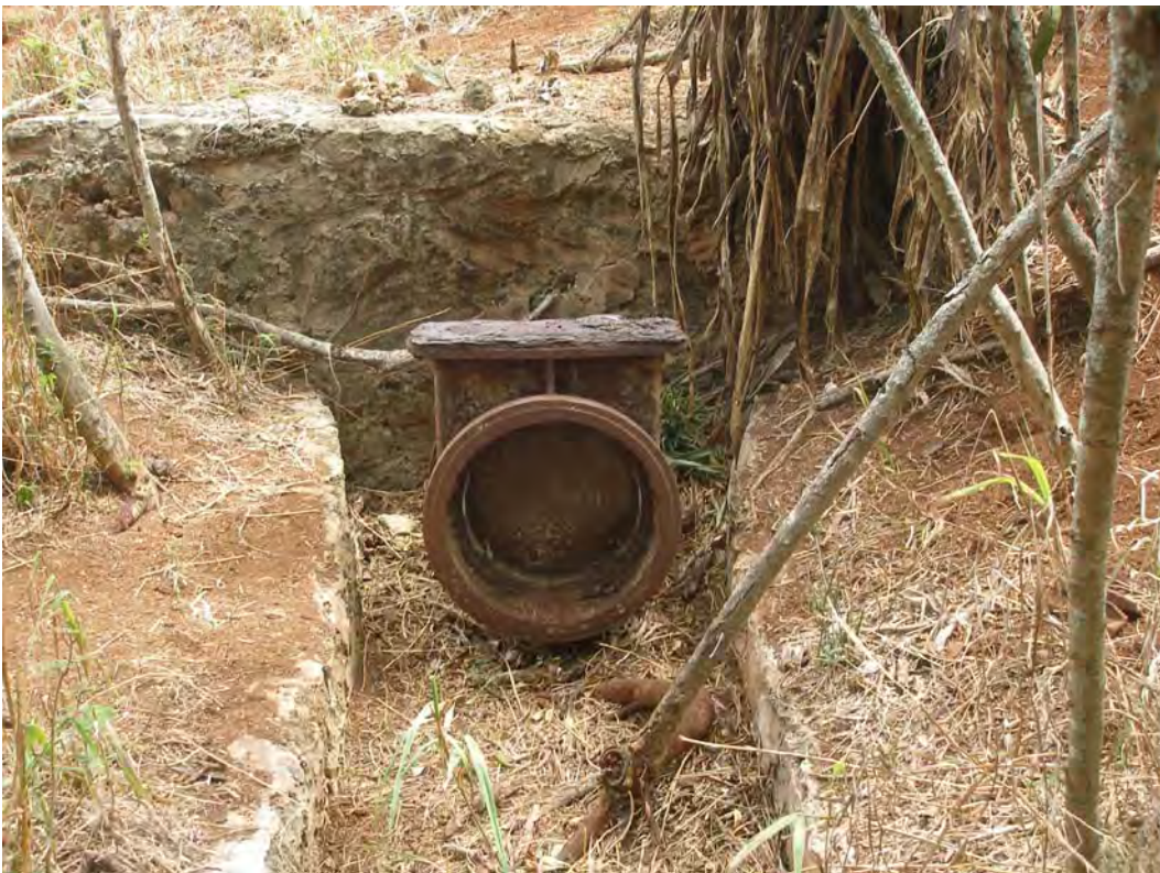
Figure 36. Reservoir inlet pipe/valve, view to north.
