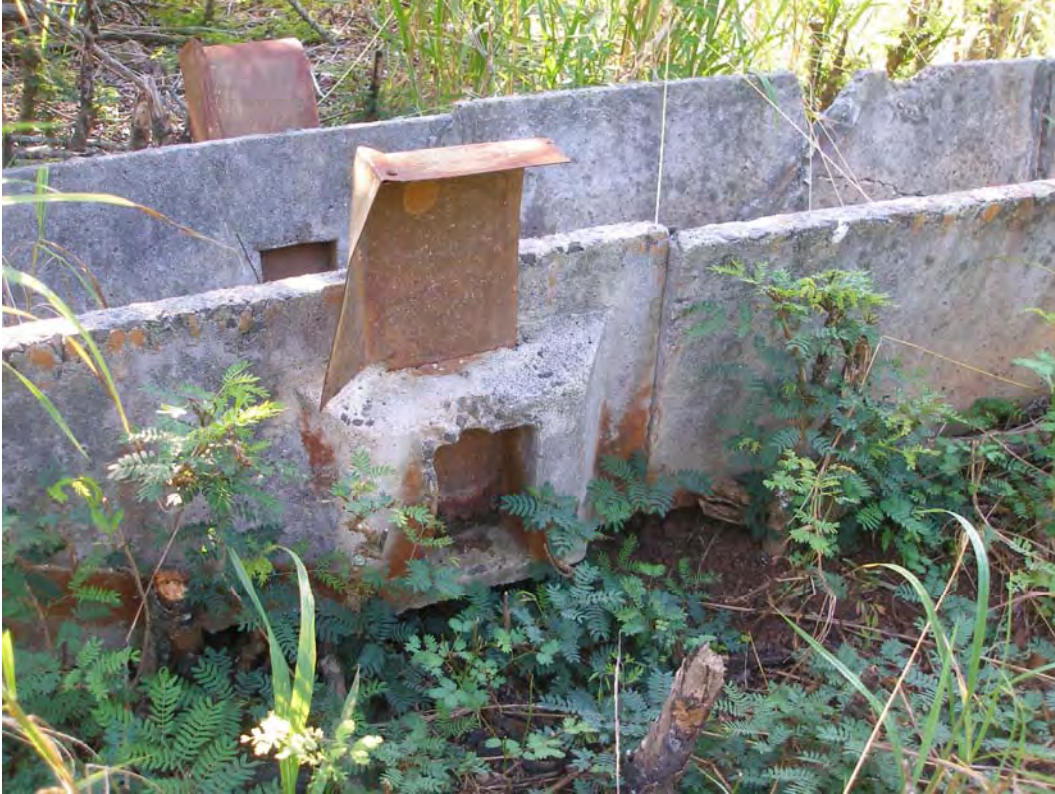
Figure 28. Sectional concrete flume Type 2 outflow opening.
