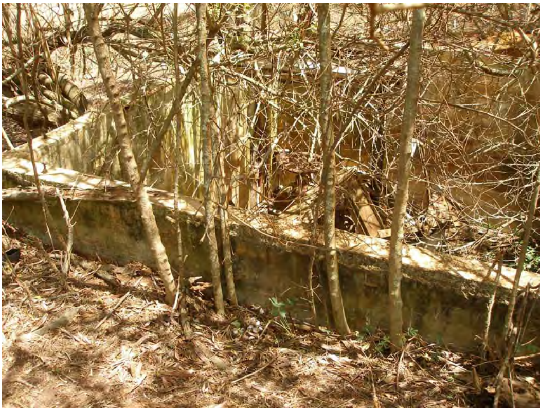
Figure 46. Pump 18 foundation, view to northeast.
