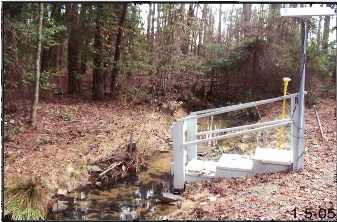
Figure 2-15. View of Outfall H-02.
