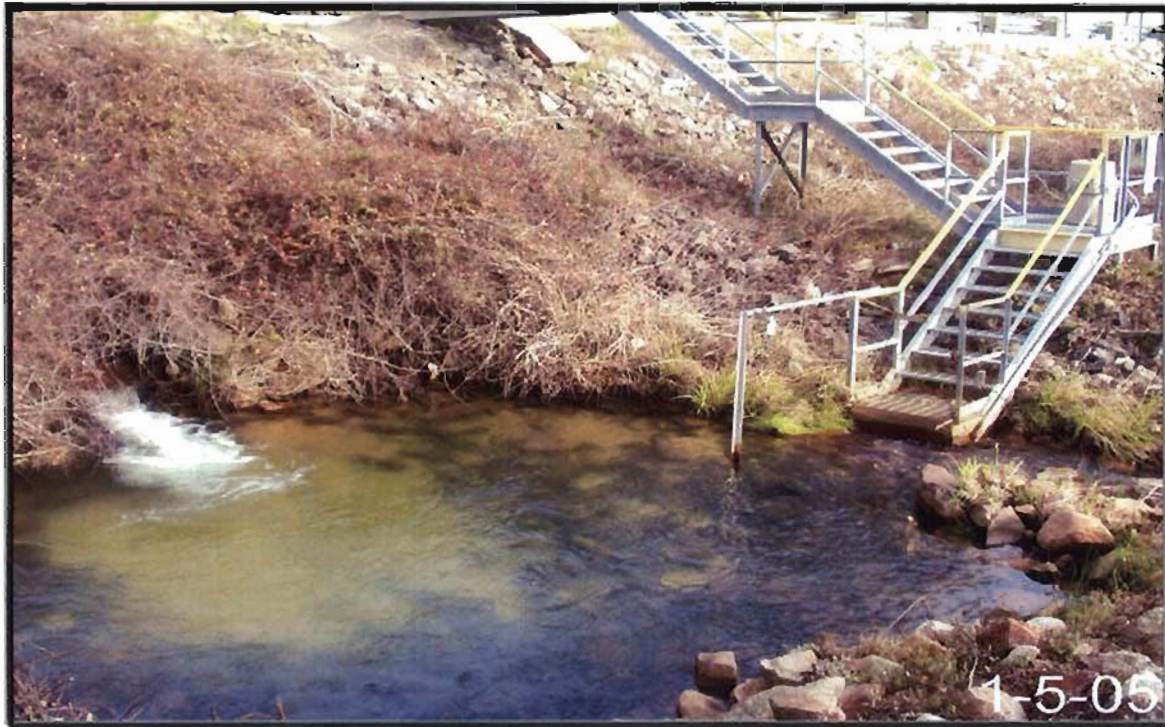
Figure 2-12. View of Existing Outfall F-08.
