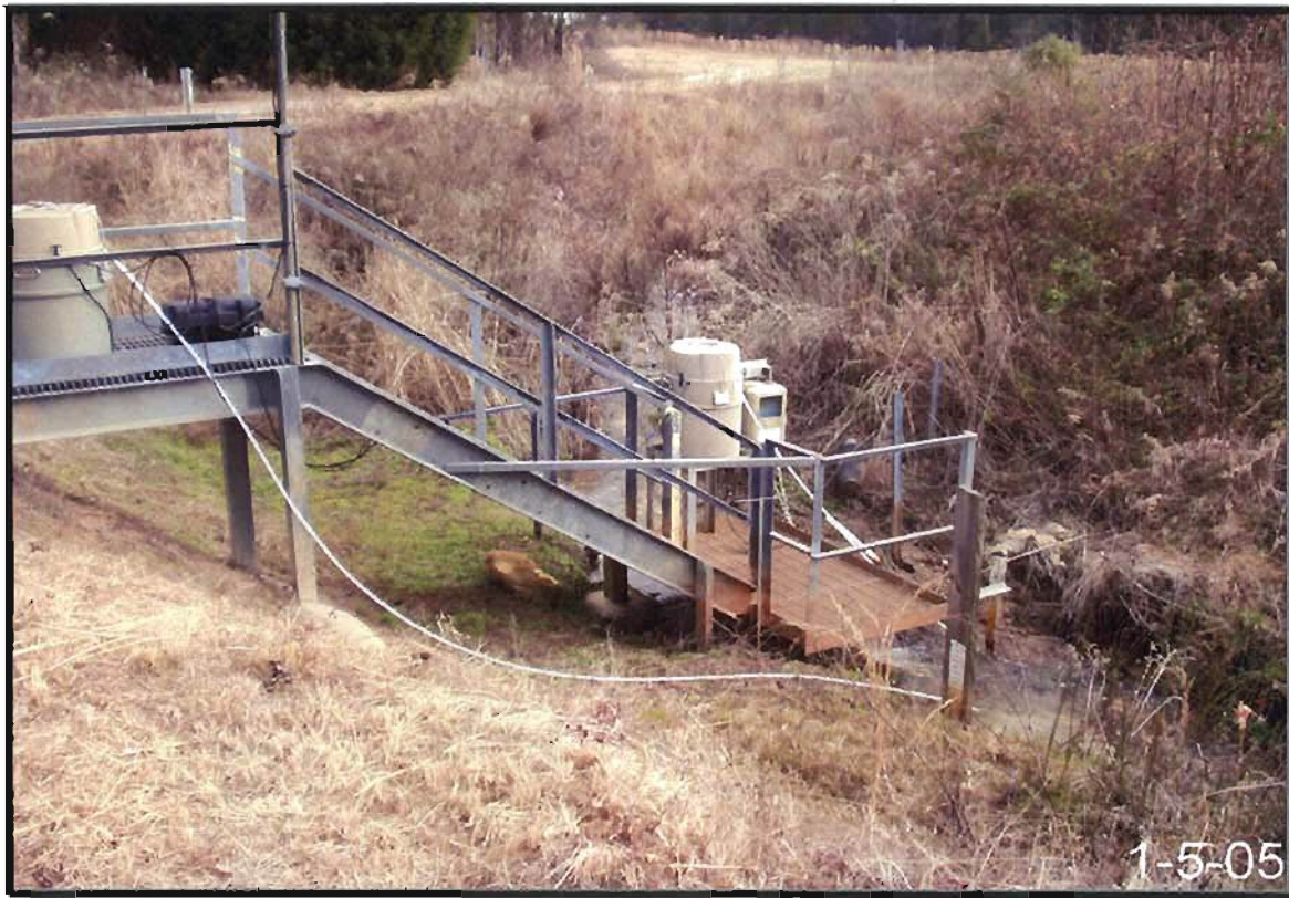
Figure 2-20. View of Outfall H-08.
