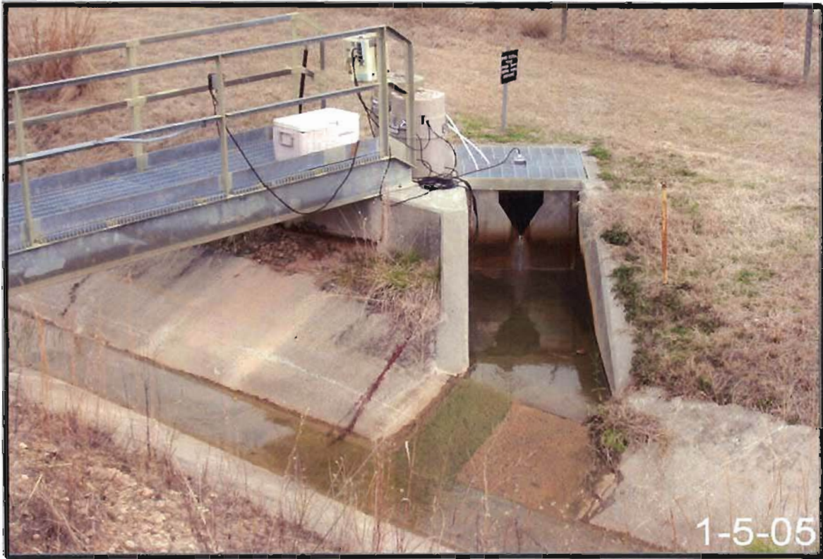
Figure 2-23. View of Outfall S-04.
