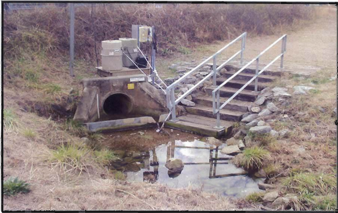
Figure 2-18. View of Outfall H-04.
