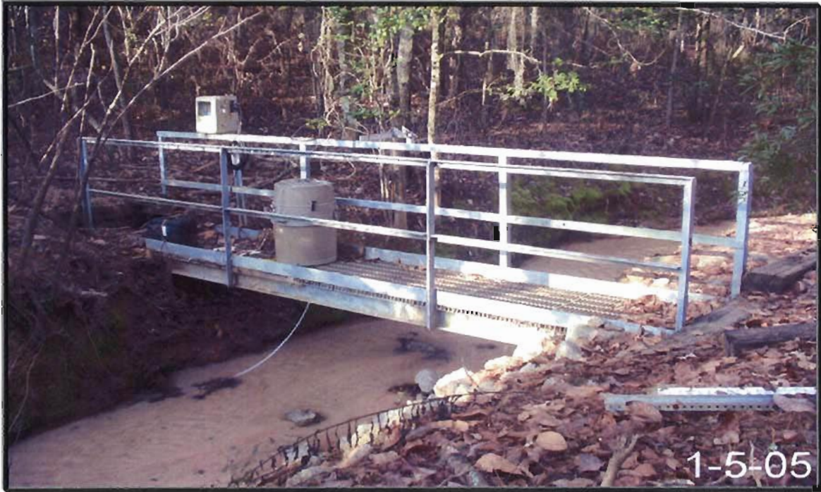
Figure 2-3. View of Outfall A-11.
