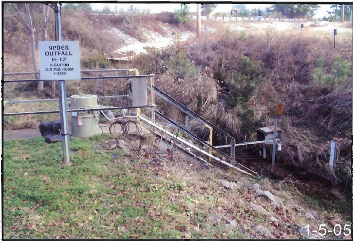
Figure 2-21. View of Outfall H-12.
