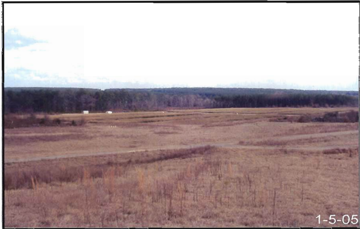
Figure 2-4. View of Constructed Wetlands Treatment Facility Downstream of Outfall A-01.
