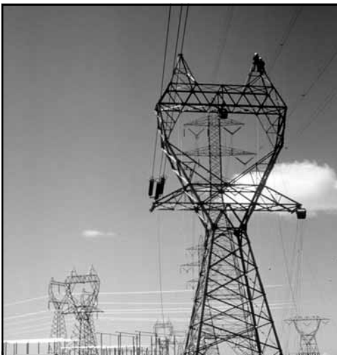
Bonneville Power Administration high-voltage energy transmission towers and power lines.
