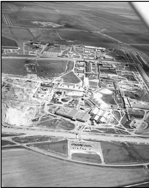
Pantex Plant—Main Production Area
