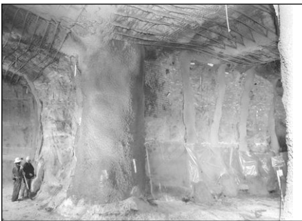
Test alcove within the Yucca Mountain repository
