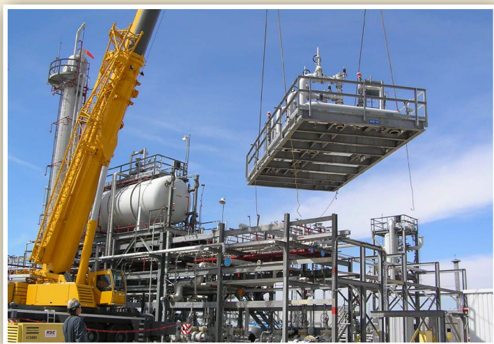
The Degas II plant being disassembled for movement to another SPR location.
