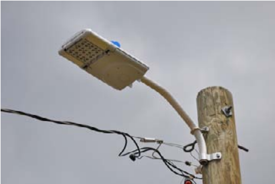
Fourteen rural towns in Utah are upgrading streetlights with LEDs. | Photo courtesy of Heber Light and Power
