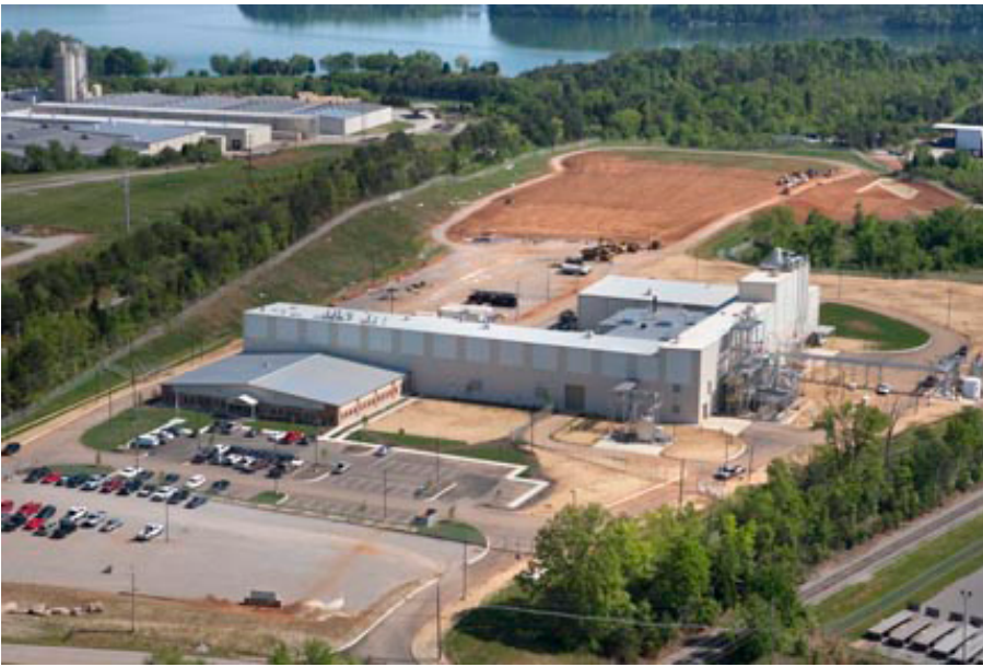
DuPont Danisco Cellulosic Ethanol (DDCE) opened a new biorefinery in Vonore, Tenn., last year. | Photo courtesy of DDCE
