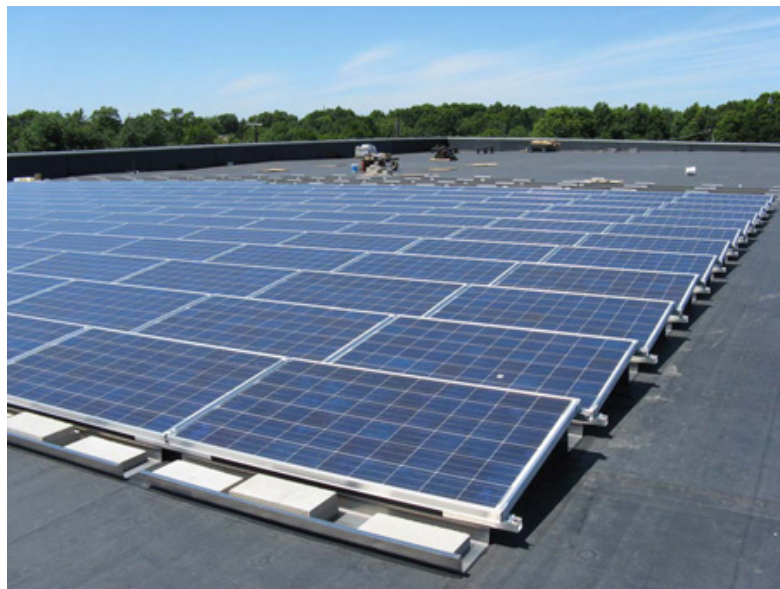
Woodbridge Township has installed solar panels atop its community center. | Photo courtesy Woodbridge
