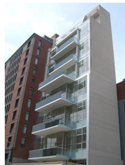
BIPV materials absorb solar energy as part of these balconies on a New York City Applied Photovoltaics project. | Photo courtesy Applied Photovoltaics
