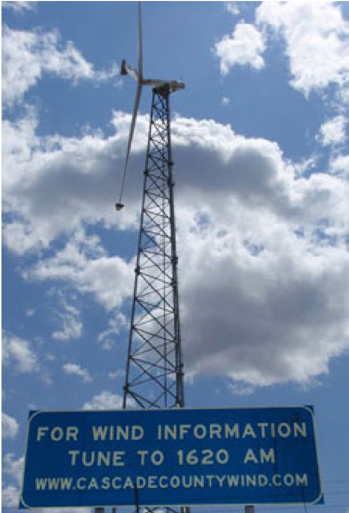
A wind turbine in Cascade County | Photo courtesy of Cascade County Commission
