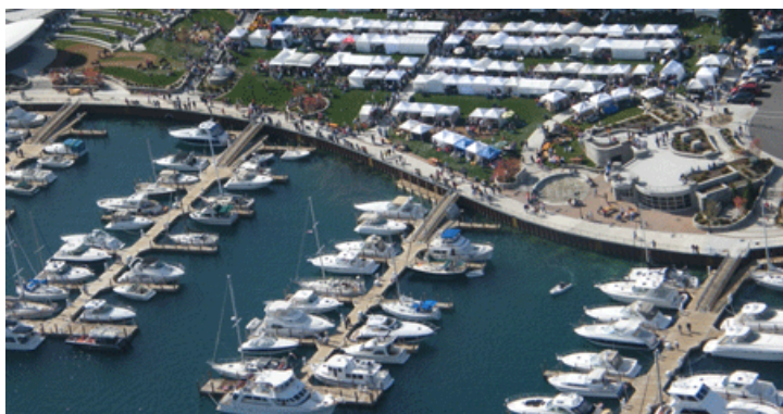
Charlevoix, Mich., is using Recovery Act funds for energy upgrades | Photo courtesy Charlevoix, Mich., city manager
