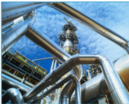
The Department has allocated Recovery Act funds to more than 25 projects that capture carbon dioxide emissions from industrial sources such as chemical plants, refineries, and manufacturing facilities, and sequester carbon dioxide into underground formations.
