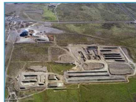
An aerial view of the F-Area at the Hanford Site in Washington State shows a wide range of waste sites during mid-cleanup activities.
