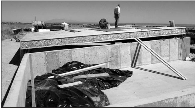
*A removable roof was constructed for a facility near the Monticello, Utah, Disposal Site that is used for temporary storage of mill tailings excavated from supplemental standards areas.*
