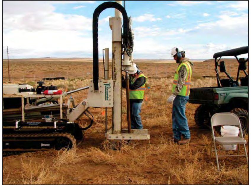
Field technicians operating a Geoprobe ® at the Highway 160 Site characterization.
