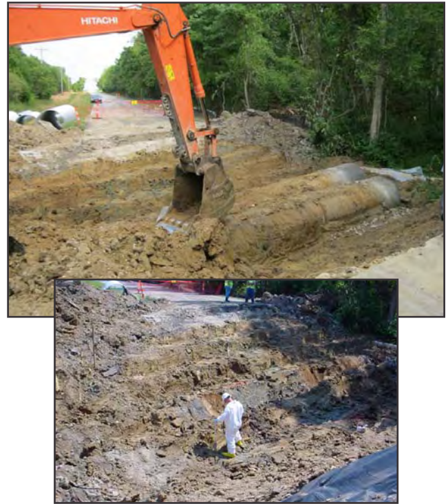
After the culverts were excavated, radiation surface scanning was conducted.
