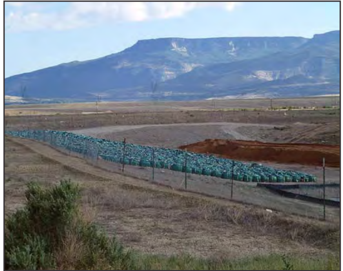
The Grand Junction Disposal Site, with loose stockpiles and bags of radiologically contaminated material from remediation of the Highway 160 Site.
