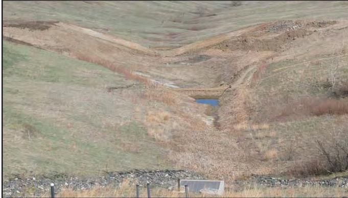
*The Present Landfill (PLF) dam breach excavation is nearly complete. In the foreground the coffer dam retains water that flows from the PLF Treatment System. Once the breach is completed, the treated water will flow into No Name Gulch.*
