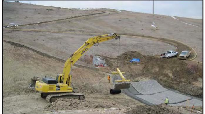
*A track hoe with boom attachment is used to place the articulated concrete armor in the dam breach channel.*
