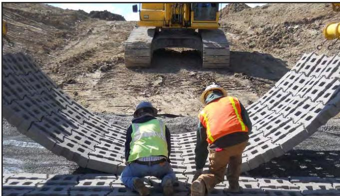
*Workers position the pieces of articulated concrete armor to provide erosion control. The concrete armor encourages the establishment of vegetation in the channel.*
