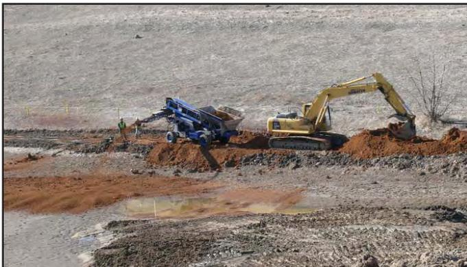
*A "soil slinger" was used in some areas to evenly fill the bowl-shaped pond bottom with soil removed during the dam excavation.*
