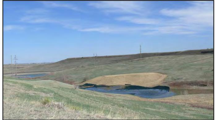
*Dam A-3 following completion. The former pond bottom has been seeded with native wetland species and the disturbed areas have been reseeded with native grasses and covered with either a spray-on mulch or erosion matting.*
