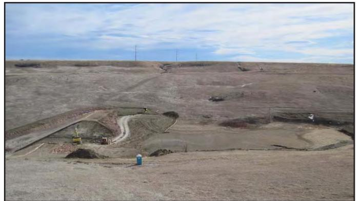
*Heavy equipment is used to excavate a notch in the dam to create a channel for surface water flow.*
