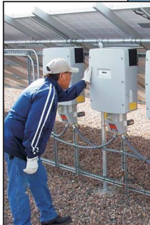
Operation of an inverter that converts solar photovoltaic DC electricity to usable AC electricity is checked regularly.
