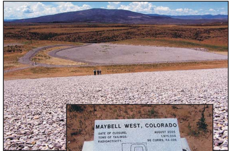
View from the disposal cell looking south toward the ancillary cell.
