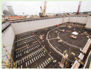
Vogtle Unit 3 Nuclear Island showing rebar installation and Containment Vessel with exterior rebar installed (Courtesy of Southern Company)
