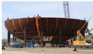
VC Summer Unit 2 Lower Bowl Assembly and Containment Vessel Ring (Courtesy of SCANA)
