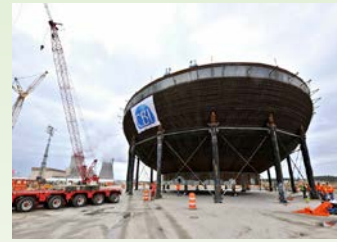
Vogtle Unit 3 Nuclear Island showing rebar installation and Containment Vessel with exterior rebar installed (Courtesy of Southern Company)
