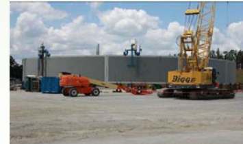
VC Summer Unit 2 Lower Bowl Assembly and Containment Vessel Ring (Courtesy of SCANA)
