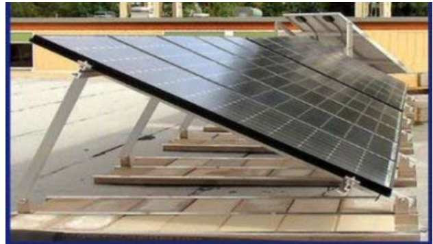
Figure 7 Ballasted PV Panels
