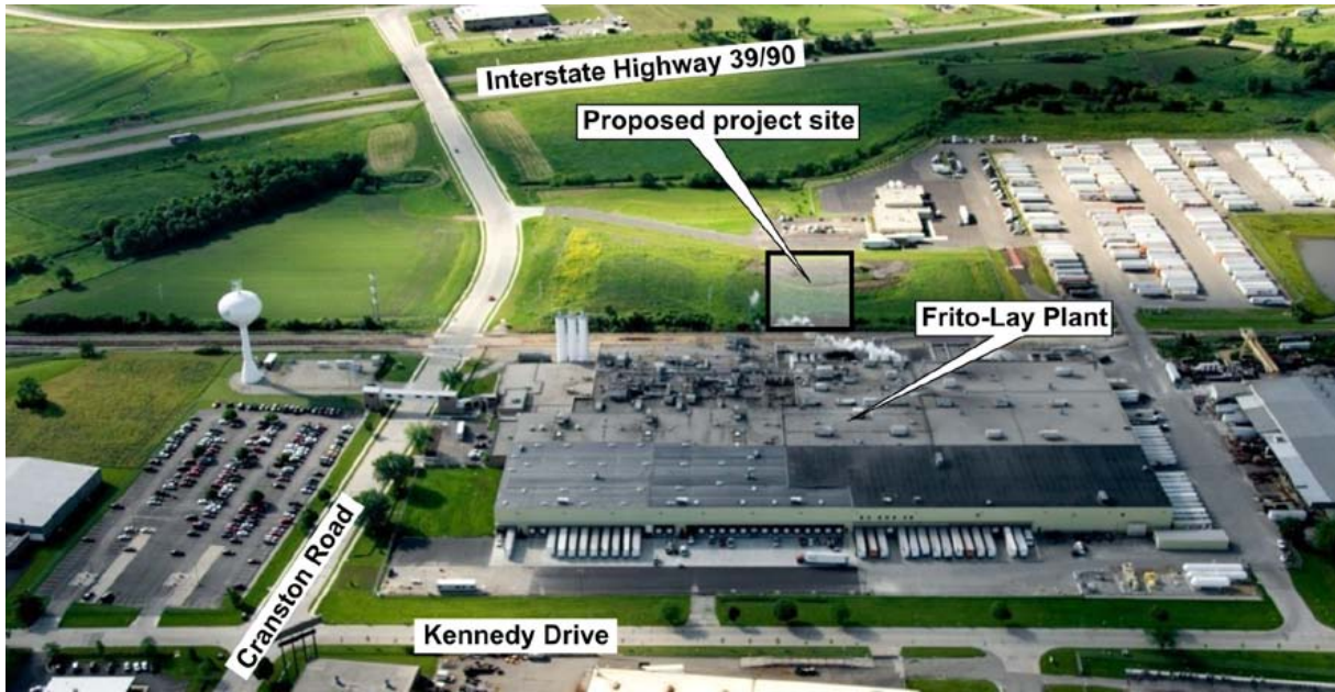
Figure 2-2. Aerial photograph of proposed project site looking southeast.
