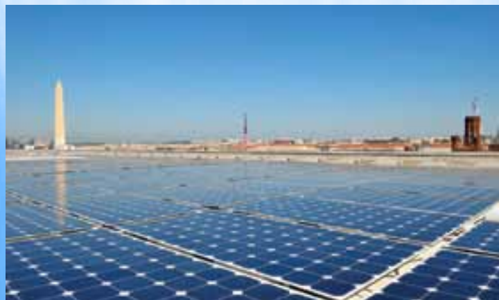
Solar roof at DOE headquarters building in Washington, D.C.
