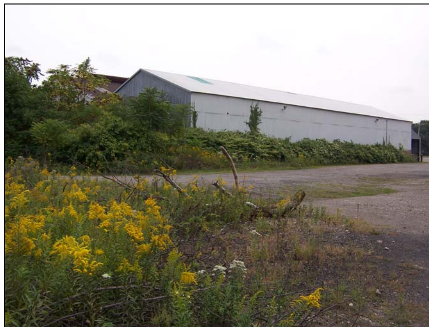
Fig. 3. Aliquippa, Pennsylvania, site, September 2005.
