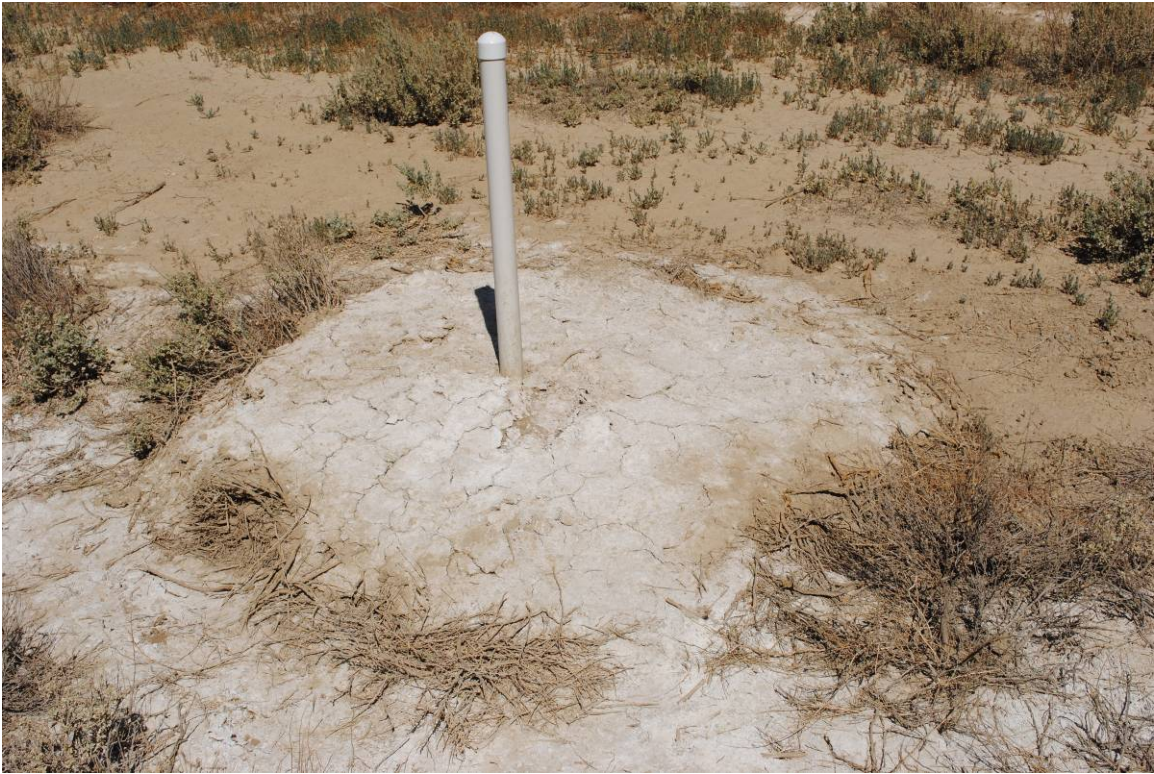
Figure 15. Sampling Point EF-19 Showing Mound Covered by Efflorescence on Ground Surface
