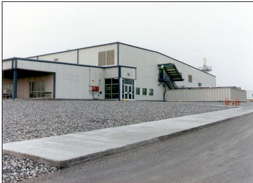
Figure S-10. Waste Receiving and Processing Facility
