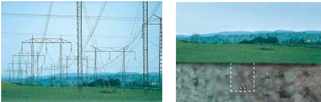
Figure 1: Overhead AC lines (left); Underground DC cables (right)
