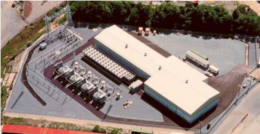
Figure 2-12 Typical Converter Station (300 MW)
