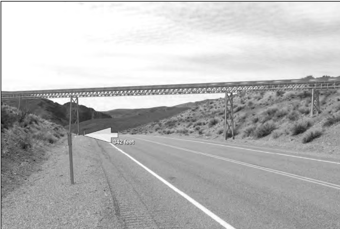
Figure D-9. Simulation of rock conveyor in view south-southwest from key observation point 4.
