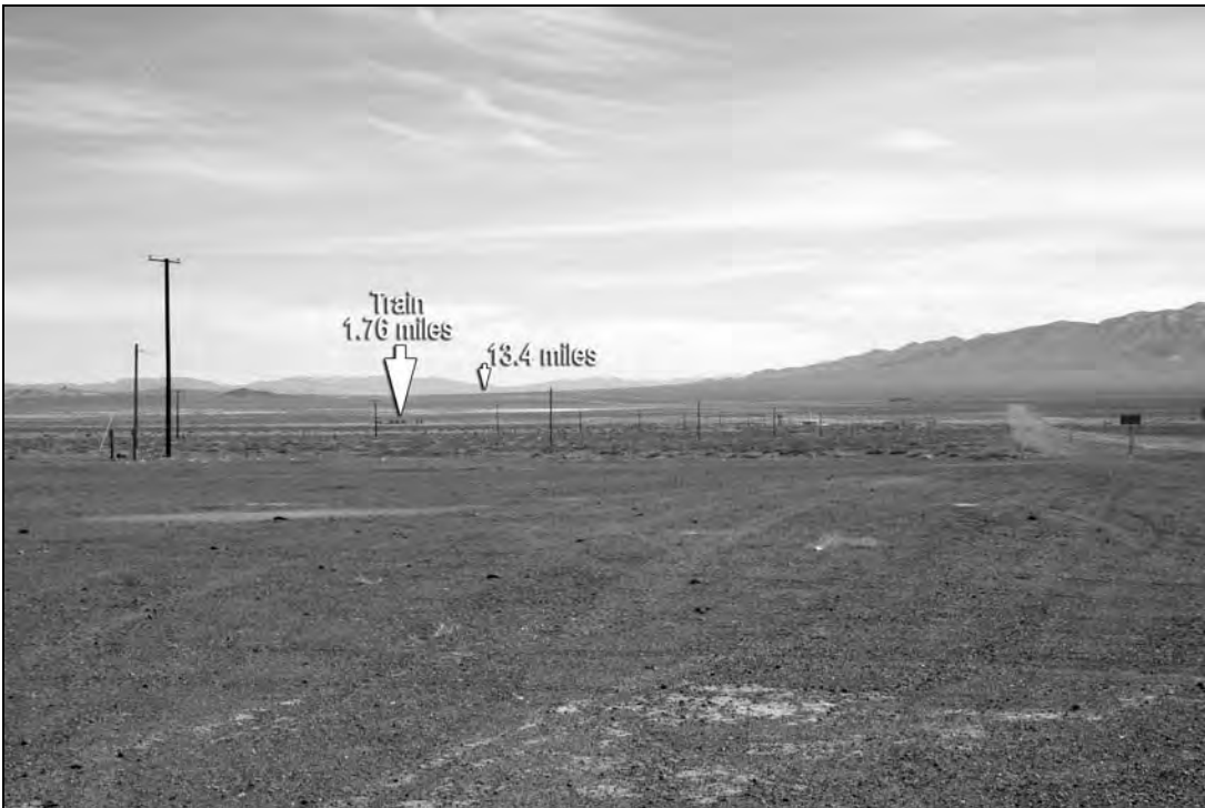
Figure D-112. Simulation of train on Montezuma alternative segment 1 running south along State Route 265 in view south-southeast from key observation point M-11 at Blair Junction.
