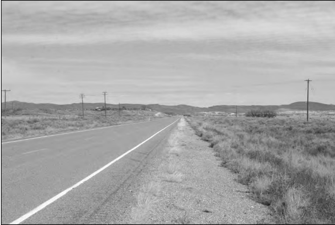
Figure D-12. View north-northeast from key observation point 6 on U.S. Highway 93 at location where rail line would cross highway.
