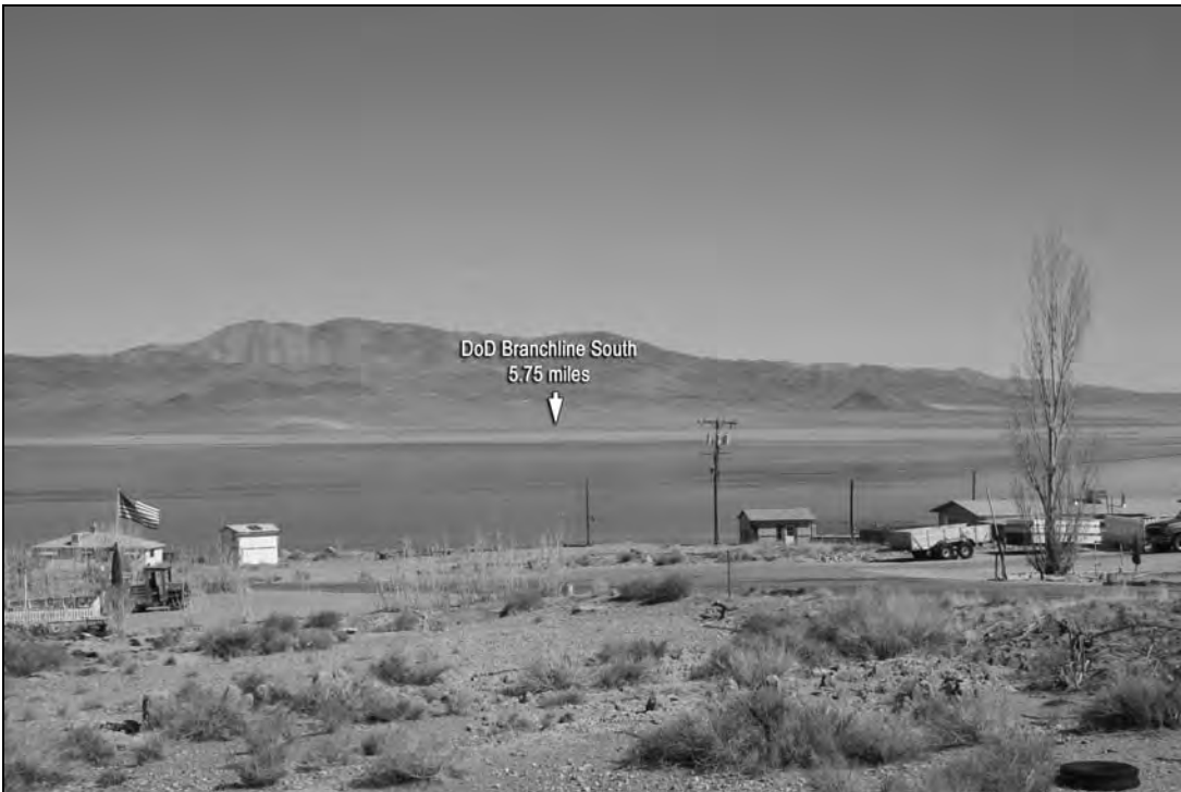
Figure D-100. View east from key observation point M-7 in the town of Walker Lake across lake toward existing Department of Defense Branchline South. Photo shows the visibility of the existing line at distance of 9.3 kilometers (5.8 miles).
