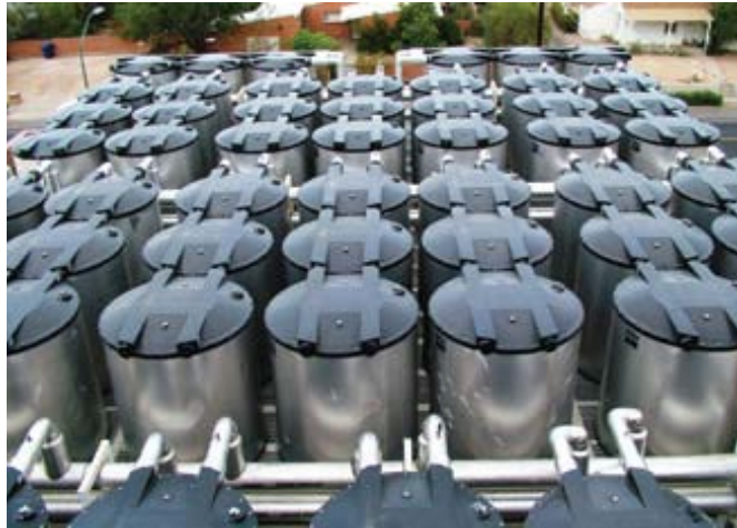
Figure 10: CALMAC Ice Storage tanks at the University of Arizona
