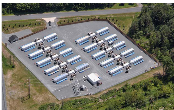
Figure 9: 20 MW Beacon Flywheel Energy Storage Plant for Frequency Regulation
