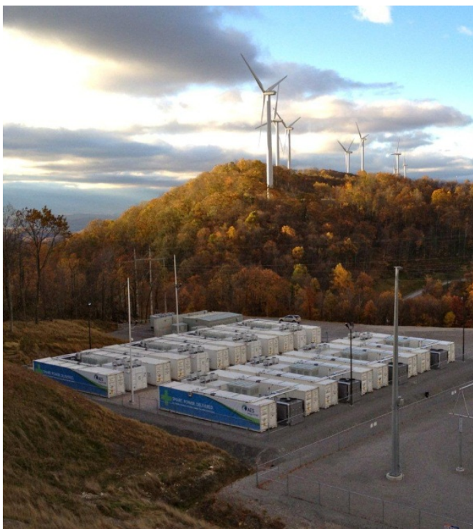
Figure 2: AES Lithium-Ion Battery Plant near a Wind Farm in West Virginia
