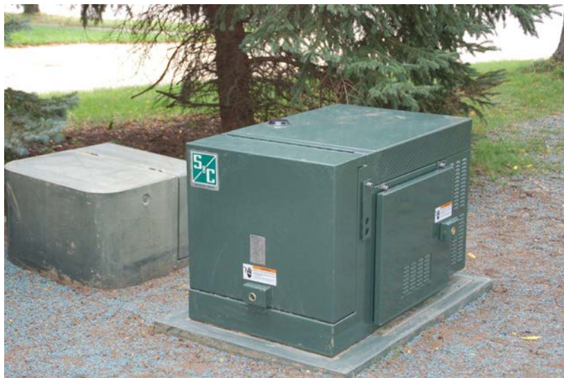
Figure 3: Community Energy Storage Unit
