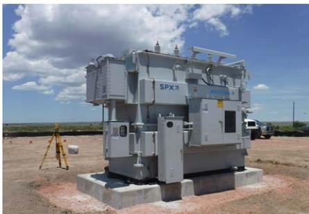
A new 20-MVA transformer installed on a foundation. As part of the new substation, it ensures power supply to the Depot campus. *Image credit: Billy Swinnea, ESG project manager for the Depot substation UESC.*
