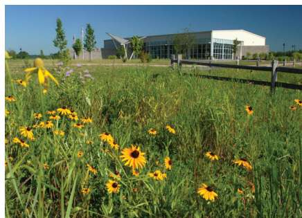
Fernald Preserve Visitors Center, Ohio
